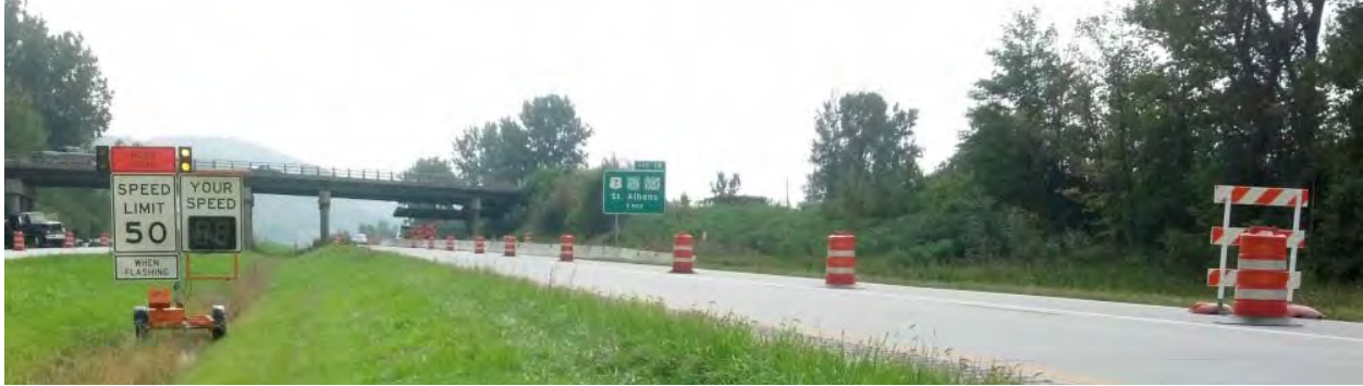
Figure 7 Saint Albans Bridge 90, Northbound RSFS
