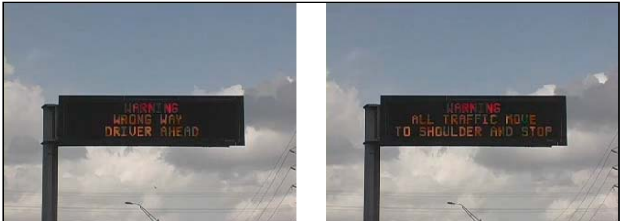
Figure 4-10. Changeable message sign (CMS) to alert right-way drivers (Thurman 2013).
