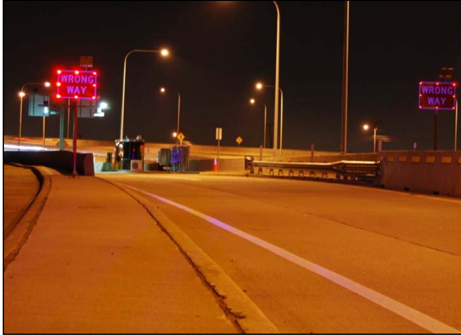
Figure 2-7. LED-enhanced WW signs (Ouyang 2013).
