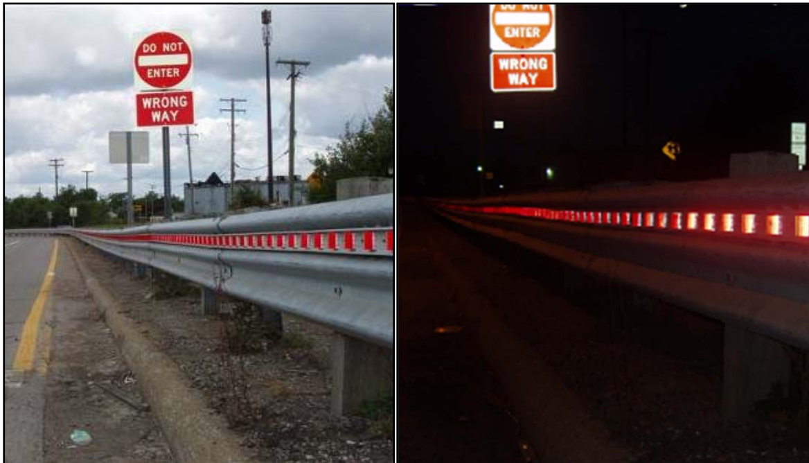
Figure 2-16. Barrier delineators visible while traveling in the wrong direction (Morena and Ault 2013).
