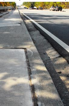
The closed flume inlet storm drain is an inconspicuous but important safety feature of the roadway.
