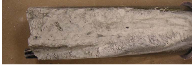
Figure 61—Top of tube injected with material C45; grout is white and hard
