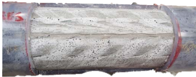
Figure 116—Segregation canal at top of cross section (PT grout)
