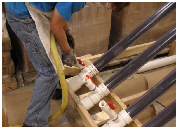
Figure 11—Attach grout hose to tube
