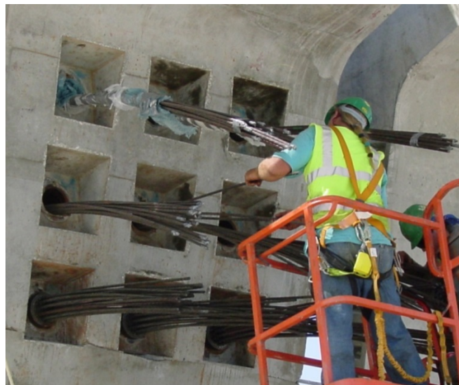
Figure 1—Precast concrete bridge segment with PT tubes and strands shown
