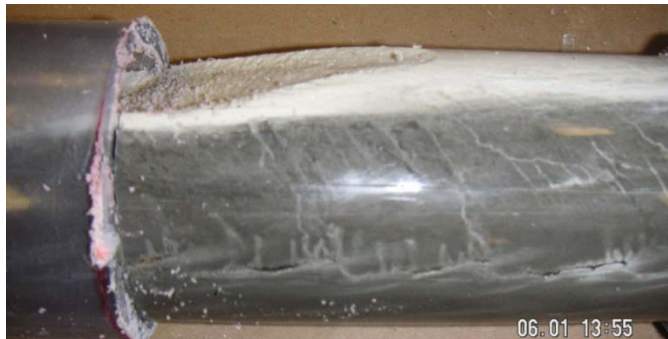
Figure 63—White grout at 12:00 position and darker grout everywhere else in tube injected with material C675
