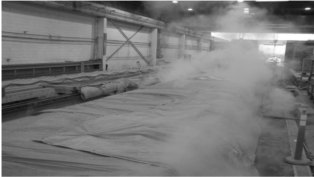
Figure 3.2 Steam Curing of Pi-Girder
