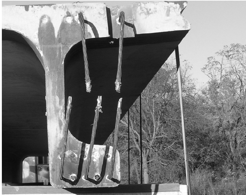
Figure 2.12-Pi-Girder Longitudinal Prestressing
