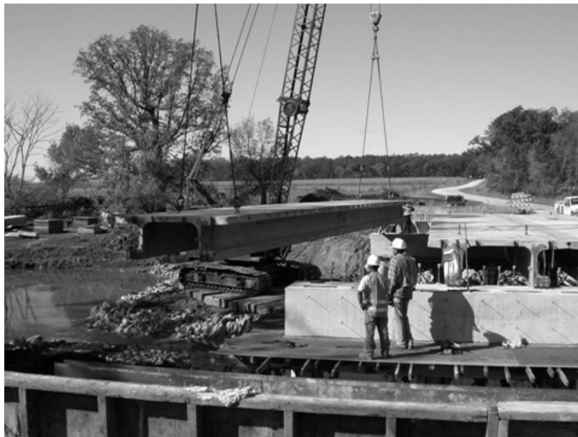
Figure 3.3 Erection of Pi-Girders
