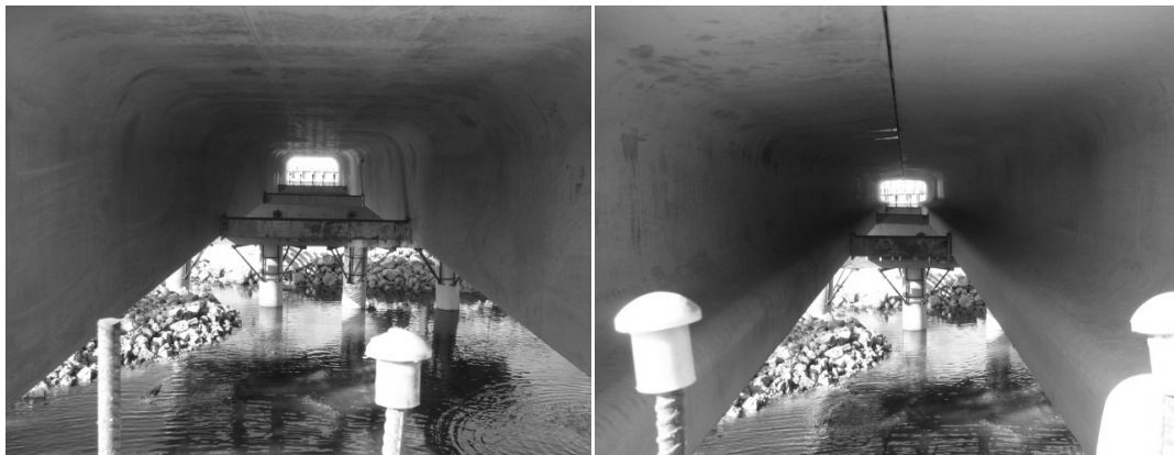
a. Diaphragm in a girder
