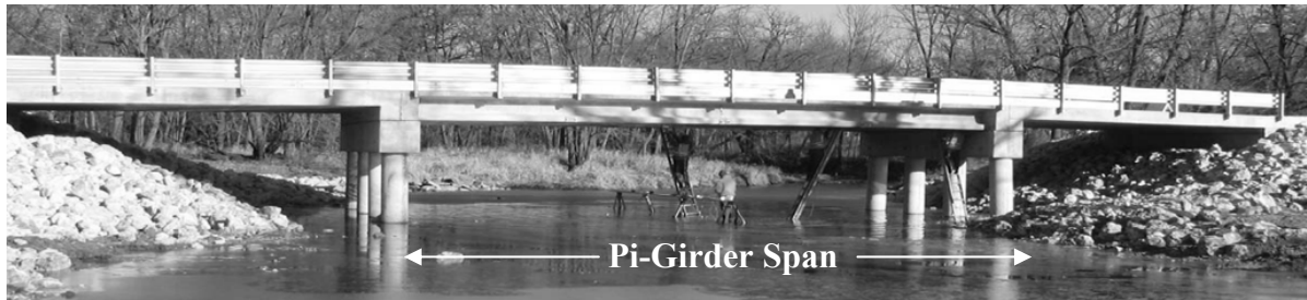
Figure 2.5-Elevation Photograph of Pi-Girder Bridge
