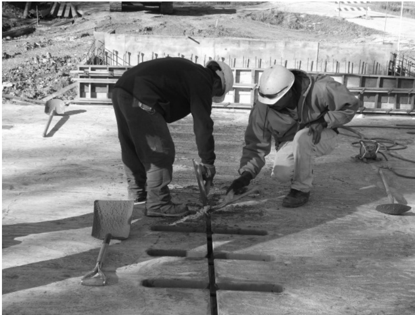
Figure 3.4 Connecting the Flanges of the Pi-Girders
