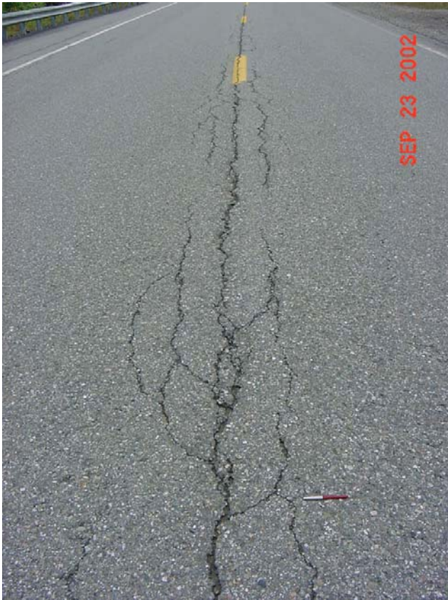
Photo 1. Control 1 Centerline Separation
