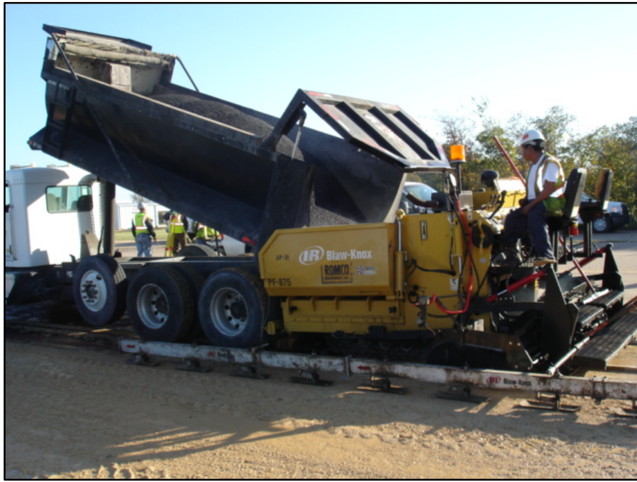
Figure 31. Paving Machine Used to Place Type C Mix.
