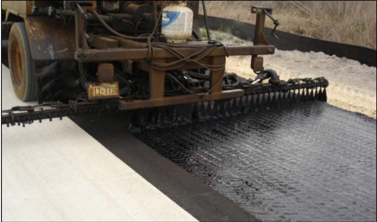
Figure 44. Asphalt Sprayed on Flexible Base for Surface Treatment.
