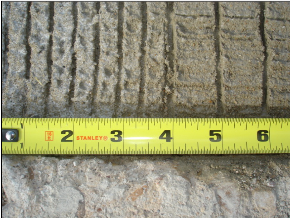
Figure 41. Change from 1/2-inch to 1-inch Transverse Tines.
