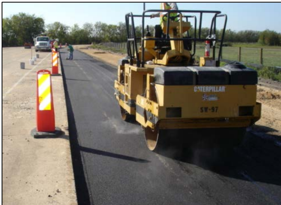
Figure 32. Steel Wheel Roller Used to Compact Type C Mix.
