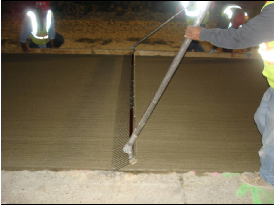
Figure 39. Concrete Surface Textured with Longitudinal Tines.
