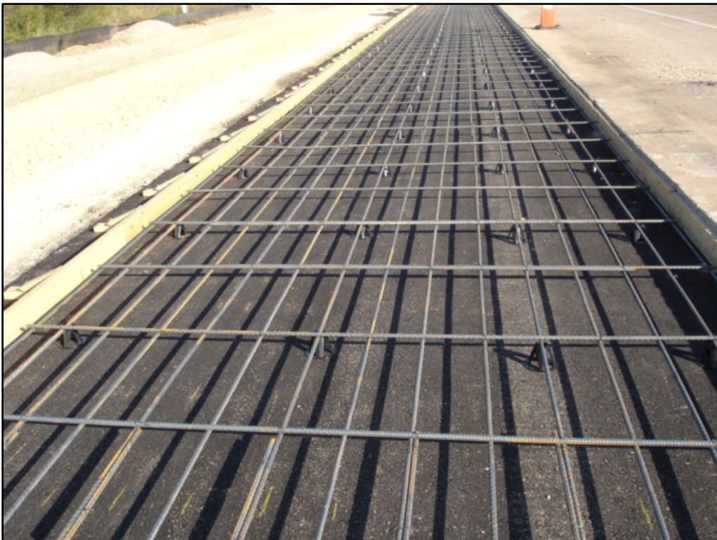
Figure 36. Reinforcement Placed for CRCP Test Track.
