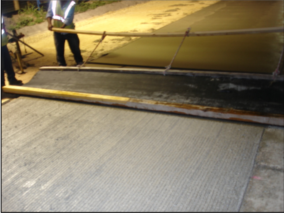
Figure 38. Concrete Surface Textured with Carpet Drag.
