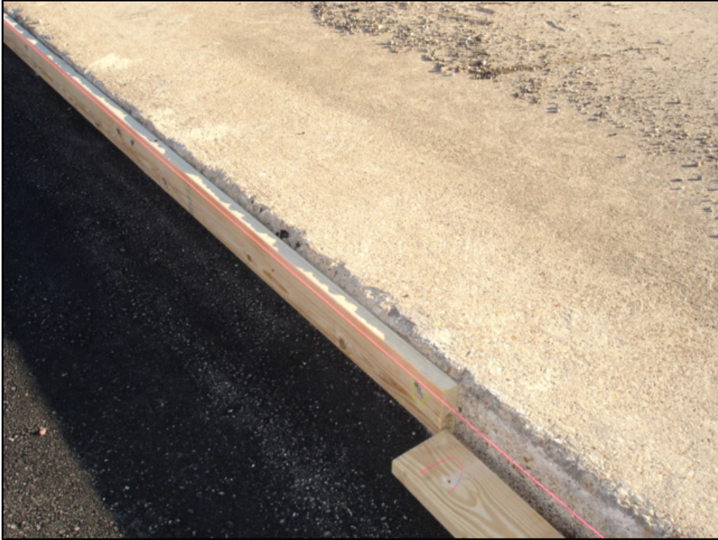
Figure 35. Placement of Form along East Side of Type C Base.
