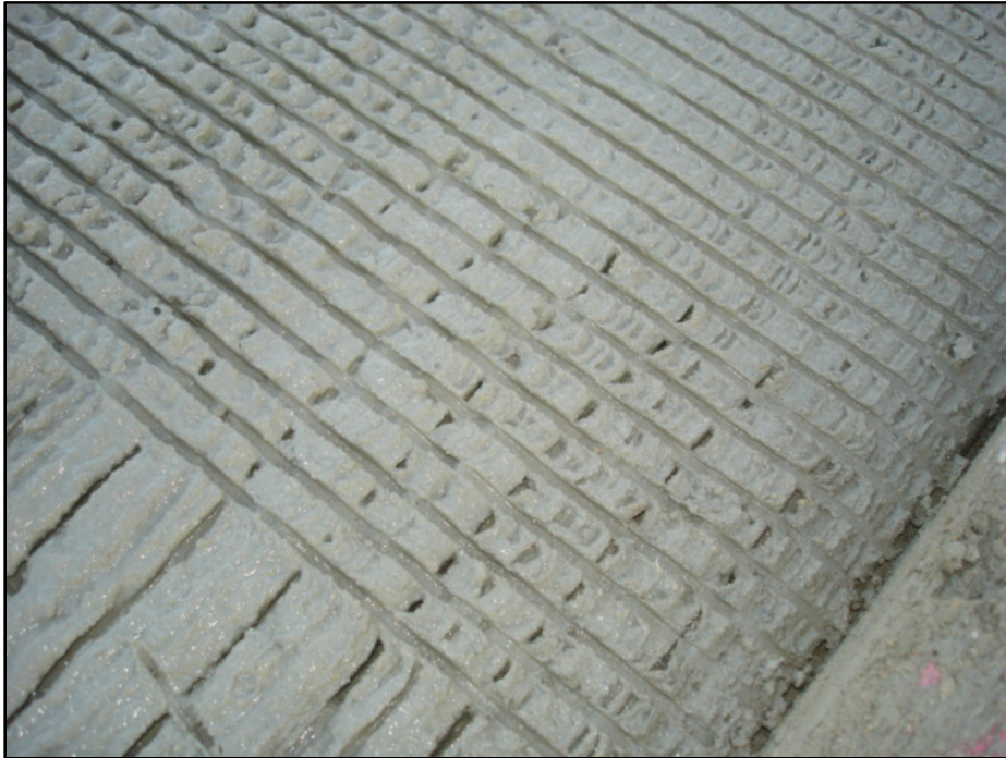
Figure 40. Change from Longitudinal Tines to 1/2-inch Transverse Tines.
