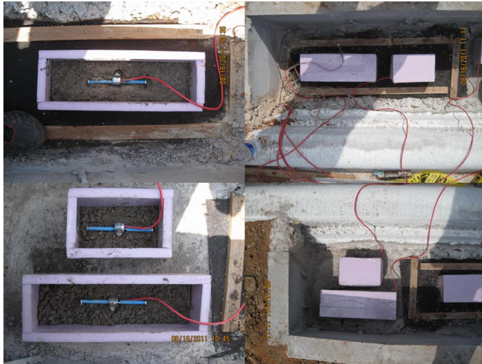
Figure 54. Concrete Prisms Cast at Field.
