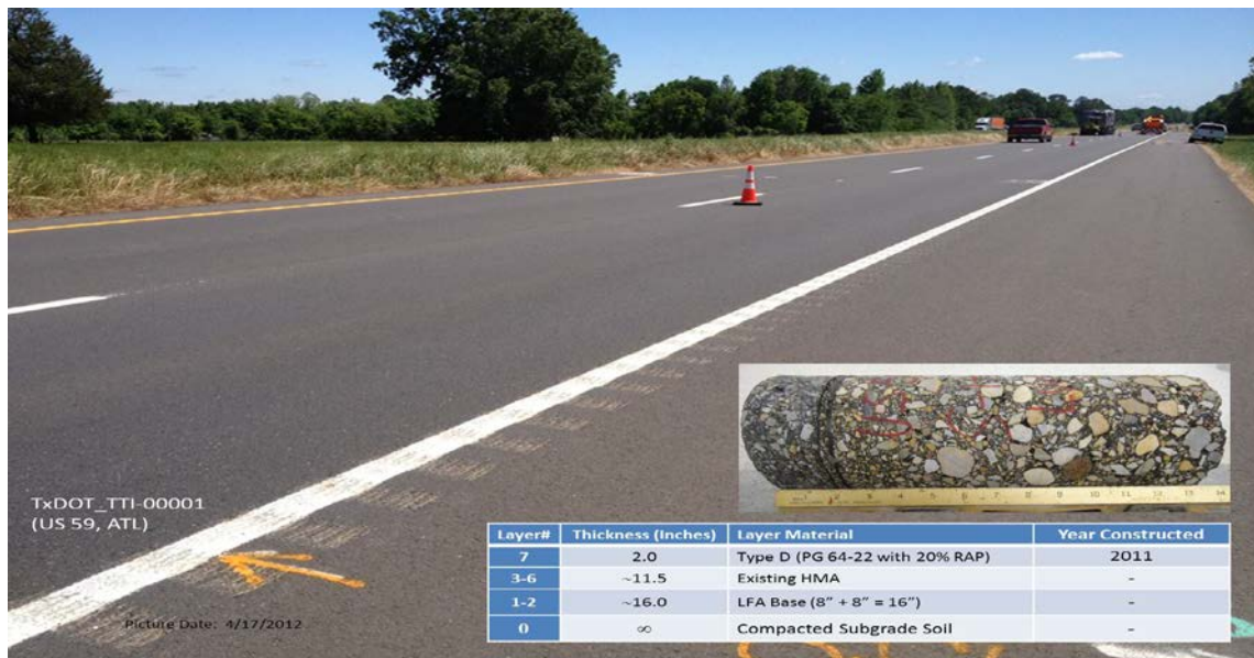
Figure 3-2. US 59 Pavement Structure in Atlanta District.
