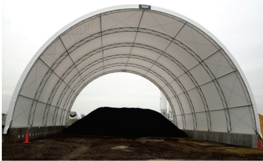
Figure 27. Covered RAS Storing Facility.
