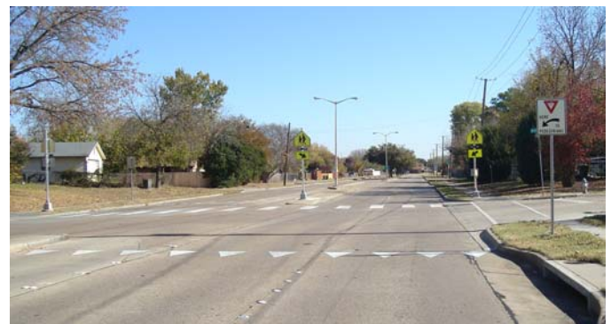
Figure 2. Example of Rectangular Rapid-Flashing Beacon Installation.
