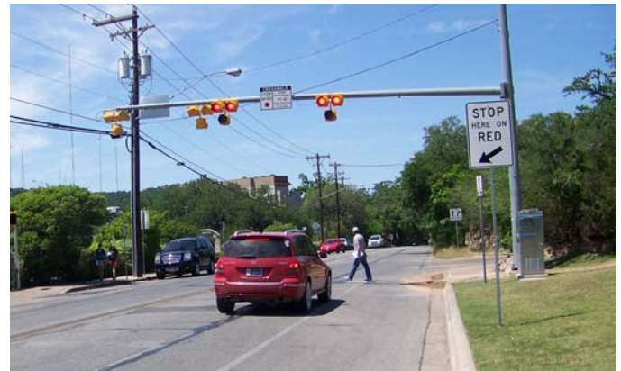
Figure 1. Example of Pedestrian Hybrid Beacon Installation.
