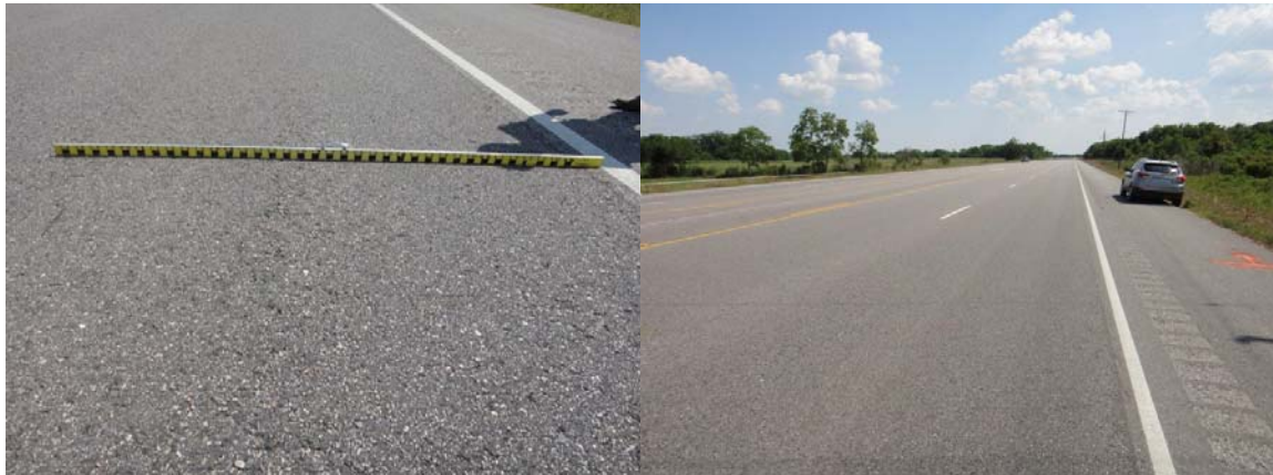
Figure 1. Good Condition of the RAP/RAS Test Section on SH 146, Houston.
