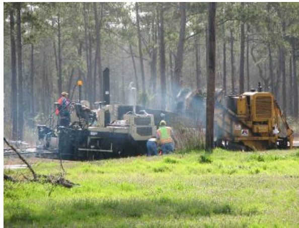
Figure 4. Construction of Lufkin WMA Field Trials.
