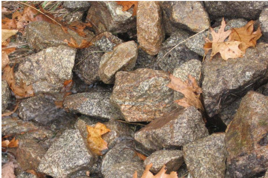
Figure 4: Outer Layer 6-8” Diameter Stone Casing for Filter Berm
