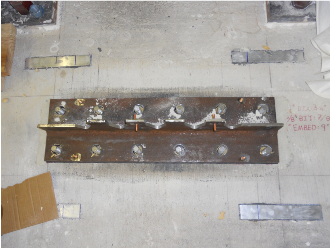
Figure D.14. Concrete anchors installed.
