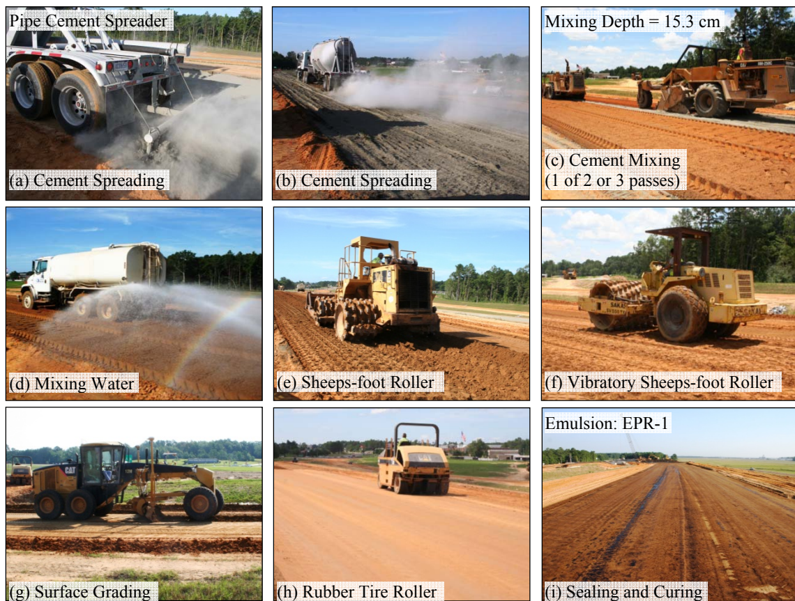
Figure 3.7. Soil-Cement Base Course Construction on State Route 475 (June 2012)
