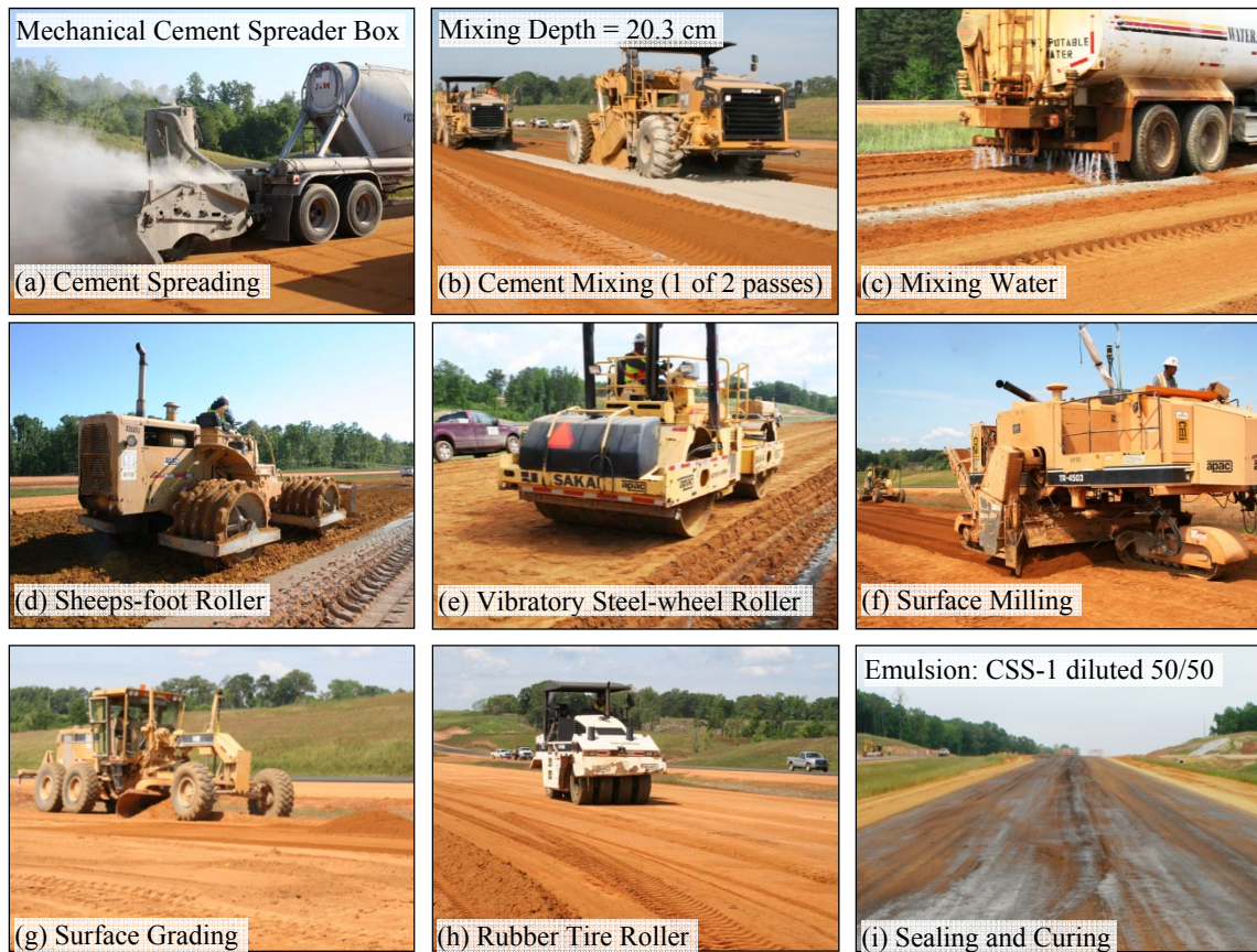
Figure 3.6. Soil-Cement Base Course Construction on State Route 9 (April 2012)
