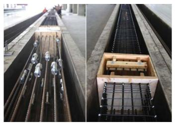
Left: a pile being constructed using steel prestressing strands. Right: a pile being constructed using CFCC prestressing strands.
