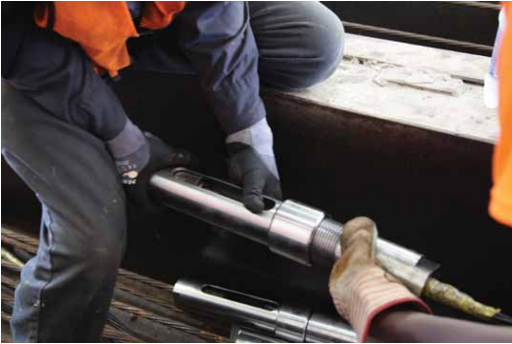
Figure H.15: CFCC coupler installation: screwing two parts together
