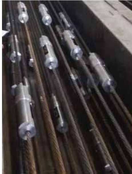
Figure 4.18: Staggered couplers after initial pretensioning
