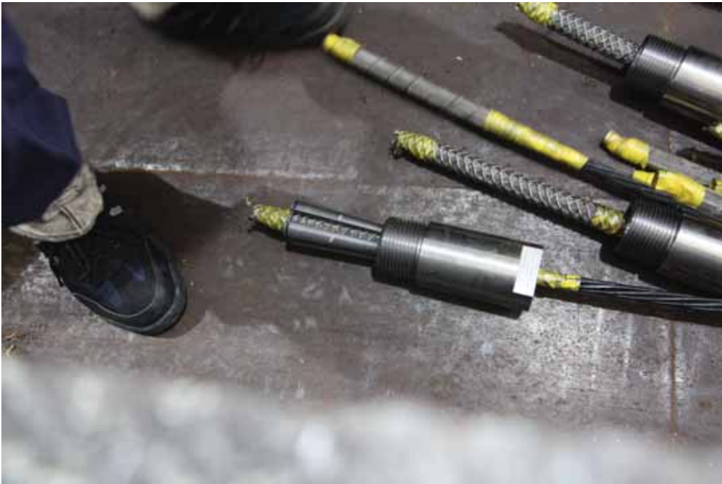
Figure H.16: CFCC coupler installation: partially-completed couplers, showing 3 stages of installation
