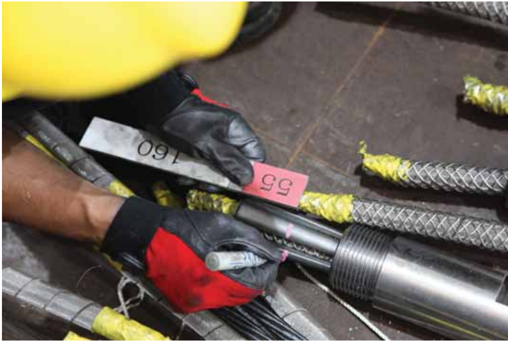
Figure H.11: CFCC coupler installation: marking wedges to prepare for pushing
