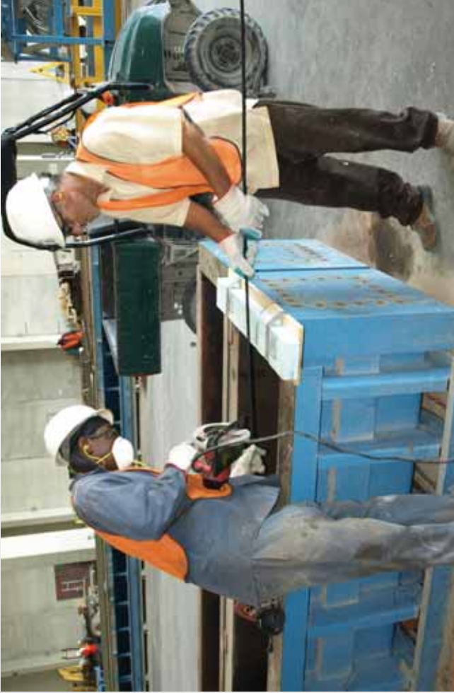
Cutting CFCC strand with circular saw
