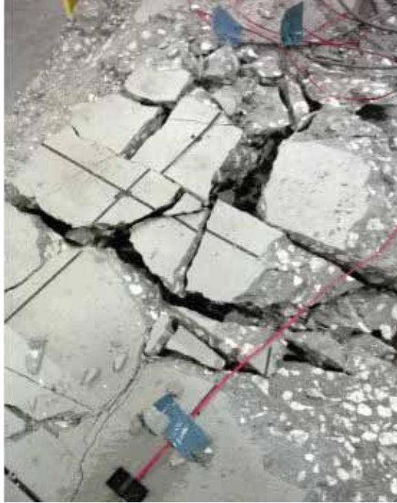
Figure 6.20: Concrete crushing at top in Test 2
