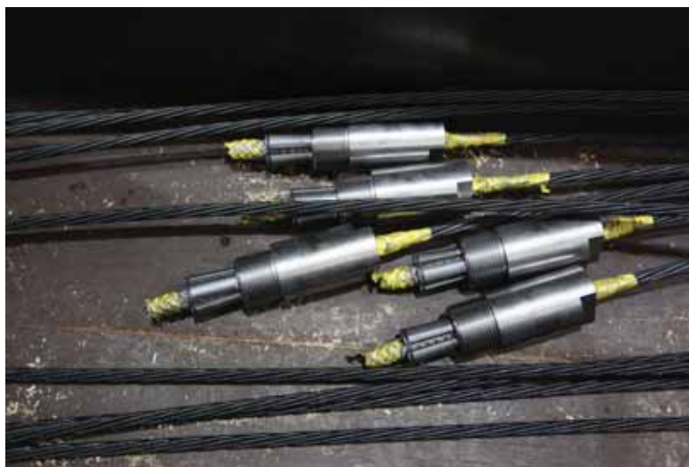
Figure H.19: Partial installation of several couplers
