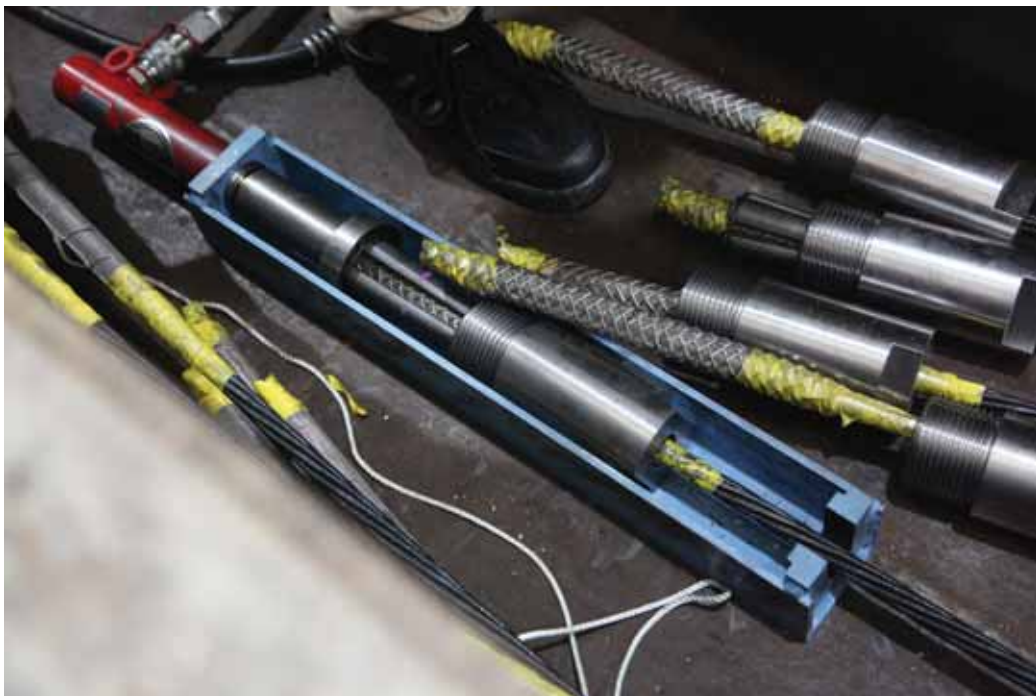
Figure H.12: CFCC coupler installation: coupler in jacking system, ready for pushing
