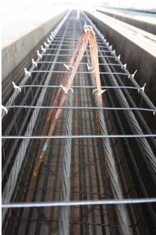
Figure H.23: Lifting loops
