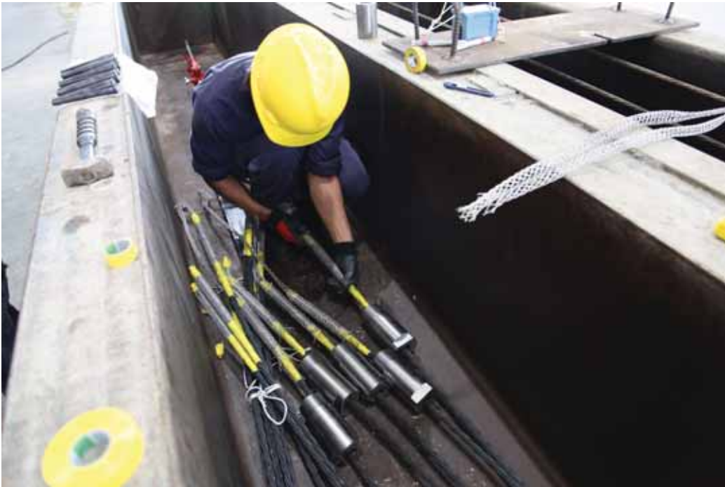
Figure H.9: CFCC coupler installation: installing braid grip on CFCC strand
