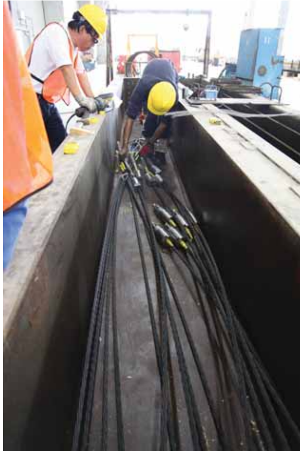
Figure H.18: CFCC coupler installation: showing several couplers in casting bed
