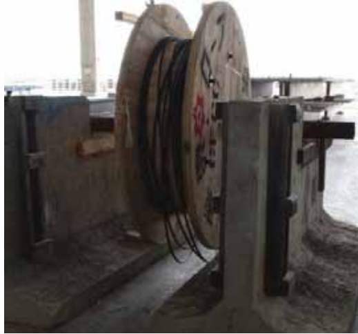
Figure 4.6: Assembly to lay strands
