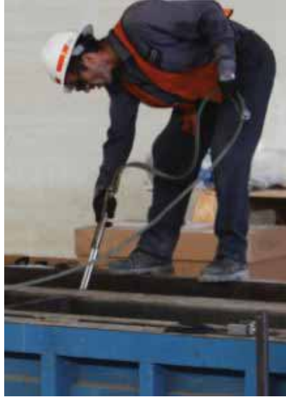
(a) Torching the steel
