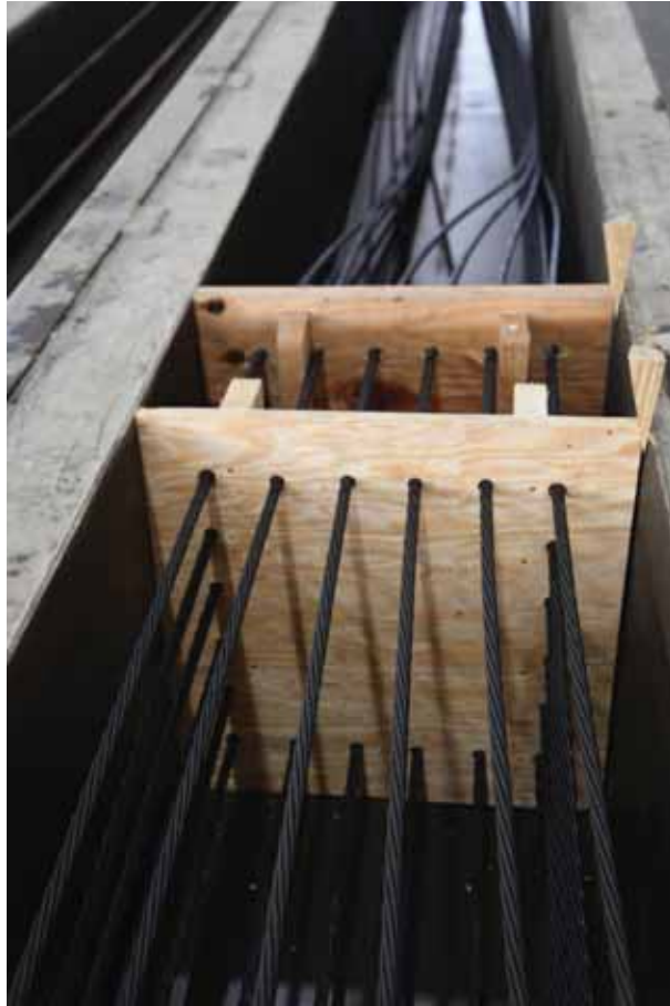
Figure H.5: Casting bed with wooden headers and installed CFCC strands
