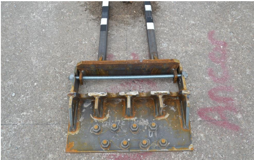
Figure 27. System Damage – Upstream Cable Anchor Bracket, Test No. HTCT-2
