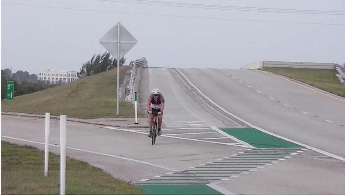
**FIGURE 6.30 Bicyclist Crossing Ramp from US 1 to Pineda Cswy Eastbound After Green Bike Lane Installation**
