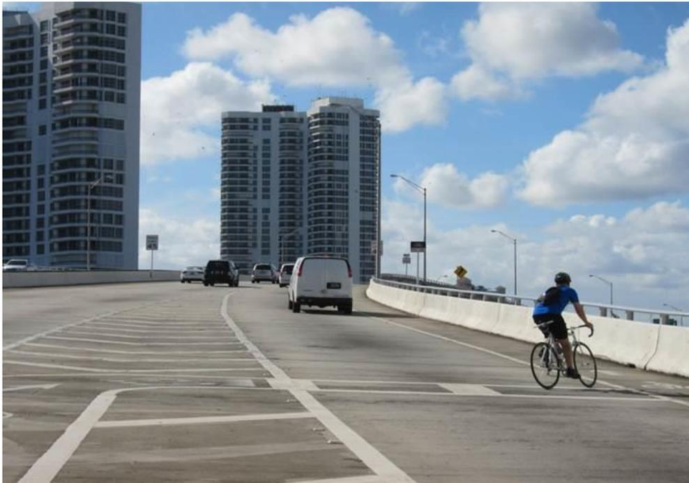
**FIGURE H.10 Bicyclist Crossing Ramp Using Bike Lane at Lehman Cswy On-Ramp**
