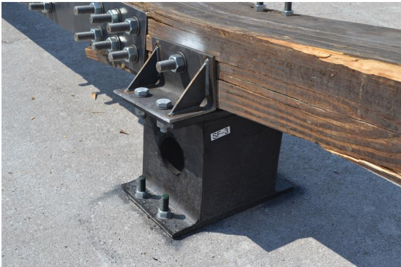
Figure 86. Post-Impact Damage, Test No. SFHT-1
