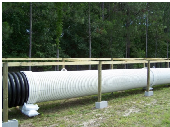
Figure 3-29: Posts with Cinderblocks
