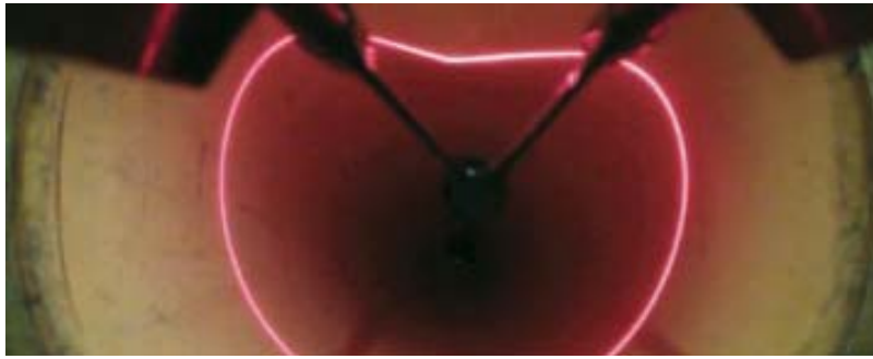
Figure 2-4: Laser Ring Profiler (from Maverick Inspection Ltd. )
