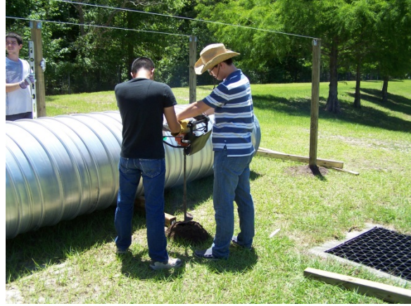
Figure 3-25: Drilling Post Holes
