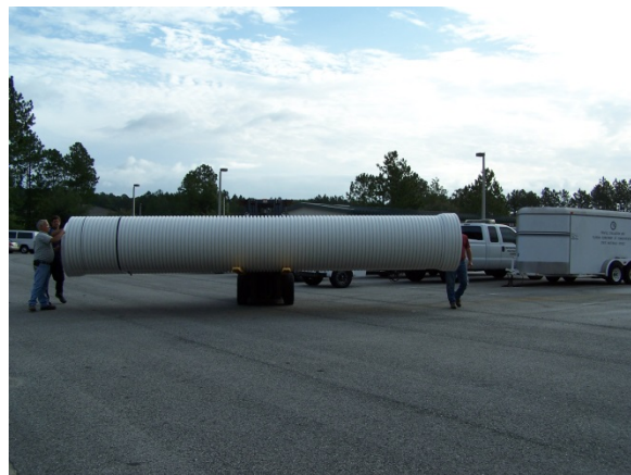
Figure 3-6: Forklift Moving PVC Pipe
