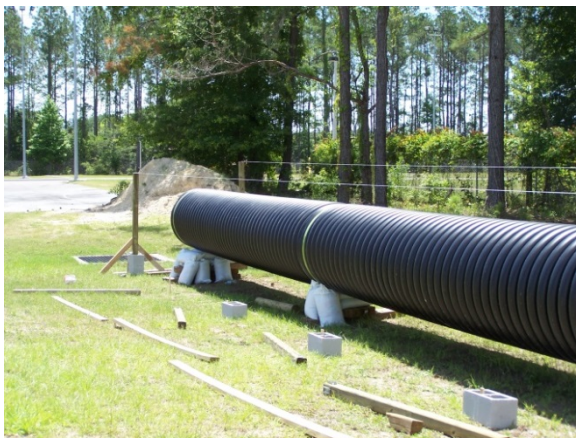
Figure 3-22: Corner Posts (East End)
