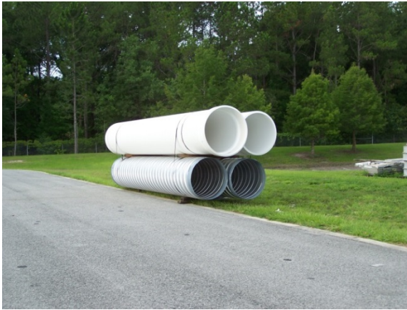
Figure 3-3: Delivery of PVC and CMP
