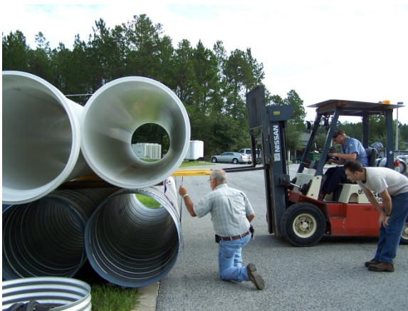
Figure 3-5: Forklift Loading PVC Pipe
