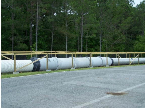
Figure 3-30: Diagonal Cross-Bracing
