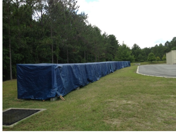
Figure 3-31: Completed Structure with Tarp
