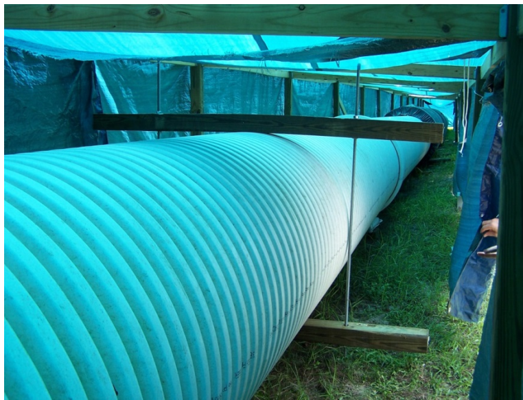
Figure 3-32: Deflection Vice on PVC Pipe
