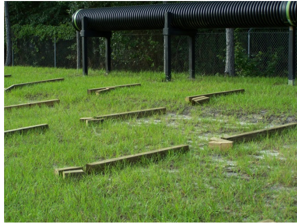
Figure 3-4: Lumber Supports and Chocks
