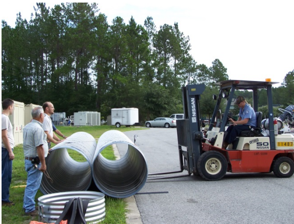
Figure 3-7: Forklift Loading CMP
