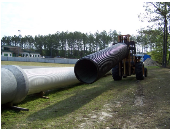
Figure 3-13: Relocating Pipe Segments
