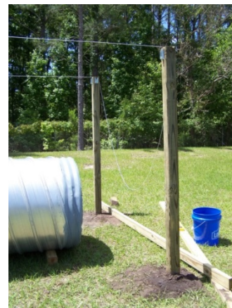
Figure 3-23: Corner Posts (West End)
