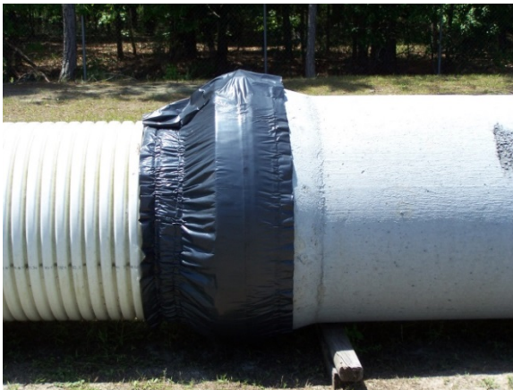
Figure 3-15: Dissimilar Pipe Coupler at PVC-to-RCP Junction
