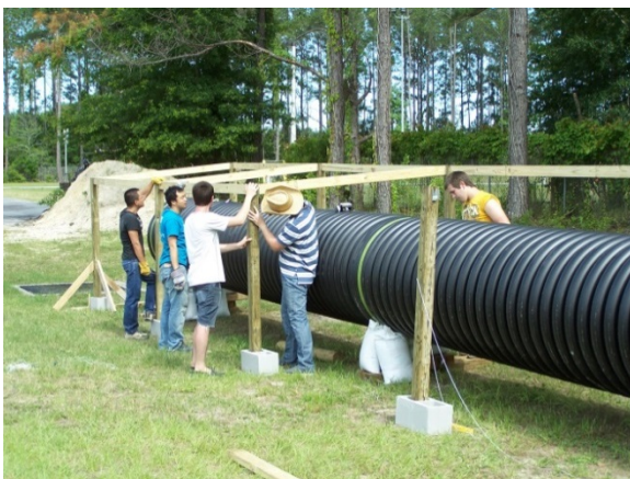
Figure 3-28: Framing Installation
