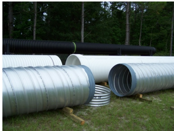
Figure 3-8: Positioned PVC and CMP
