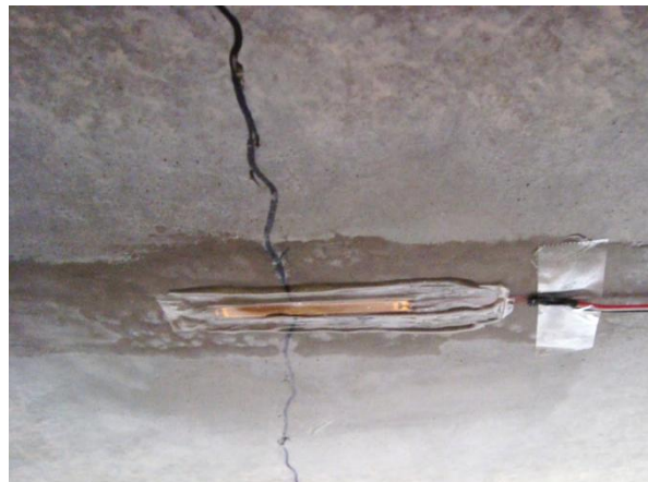
Fig. 4.4 Strain gauge attached over crack on bottom of Girder
