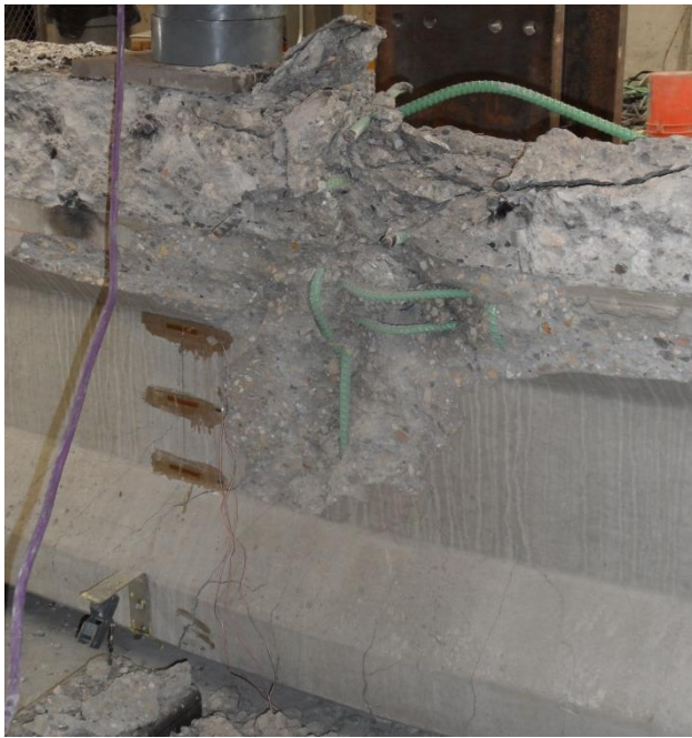
Fig. 4.21 G6-4d(b) just after concrete crushing
