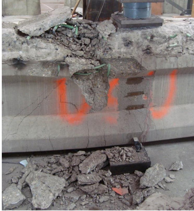
Fig. 4.10, The complete failure of the girder
