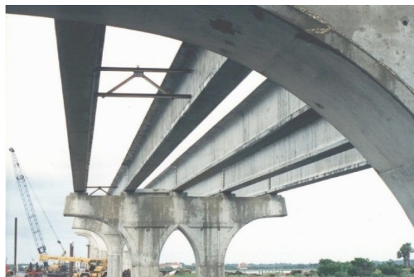
Figure 1.1 Prestressed concrete girders braced together for stability
