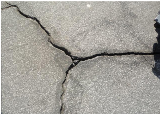
(b) Routed cracks
