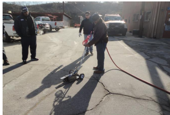
(c) Testing by GDOT crew
