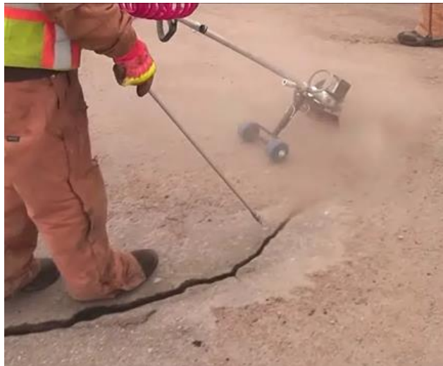
Figure 2.6 Using a detachable air wand for pavement surface cleaning by an NDOR crew
