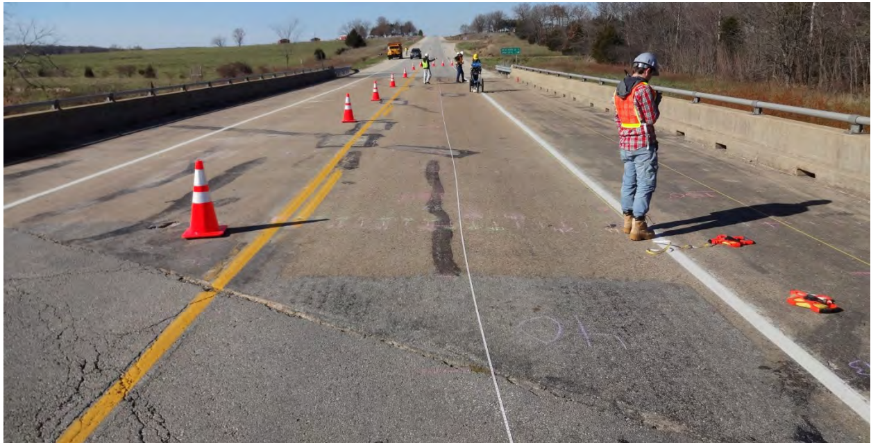
Figure 3-10 Bridge A3405 Overview of Bridge Deck Observed During Field Investigation
