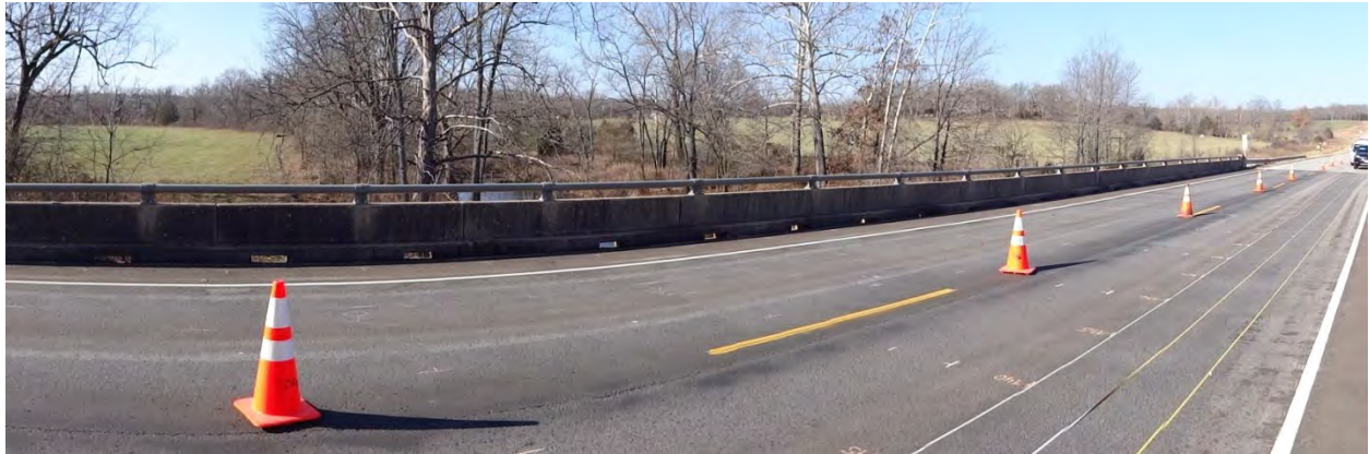
Figure 3-12 Bridge K0197 Overview of Bridge Deck Observed During Field Investigation
