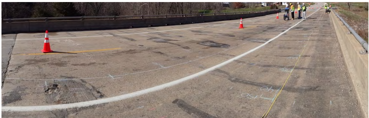
Figure 3-11 Bridge A3406 Overview of Bridge Deck Observed During Field Investigation
