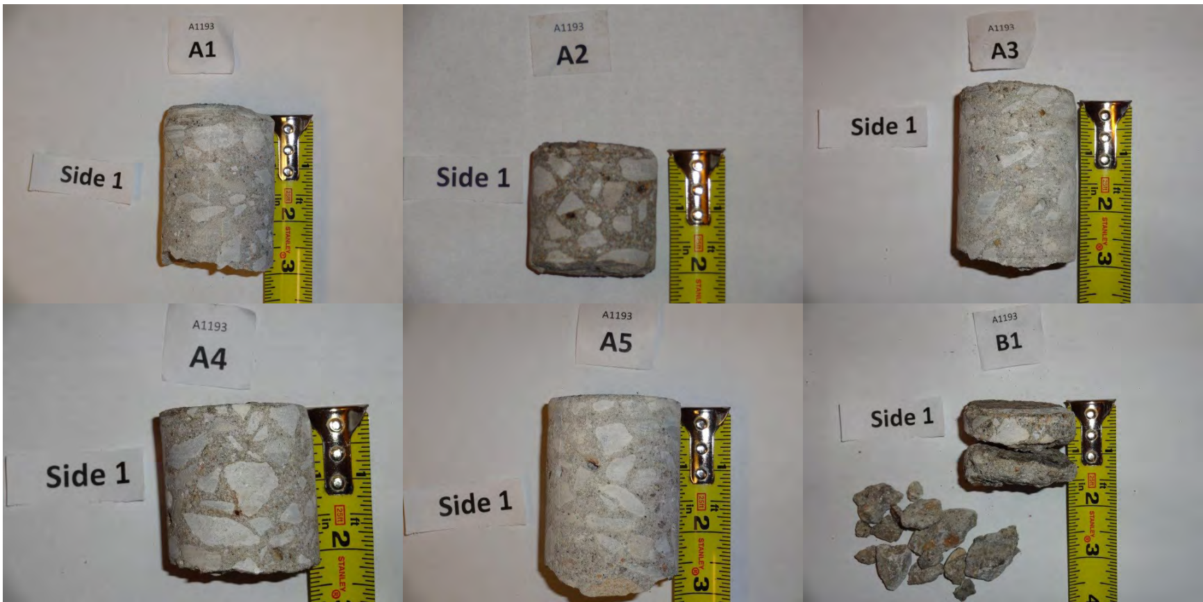
Figure 4-6 Cores Extracted From Bridge A1193
