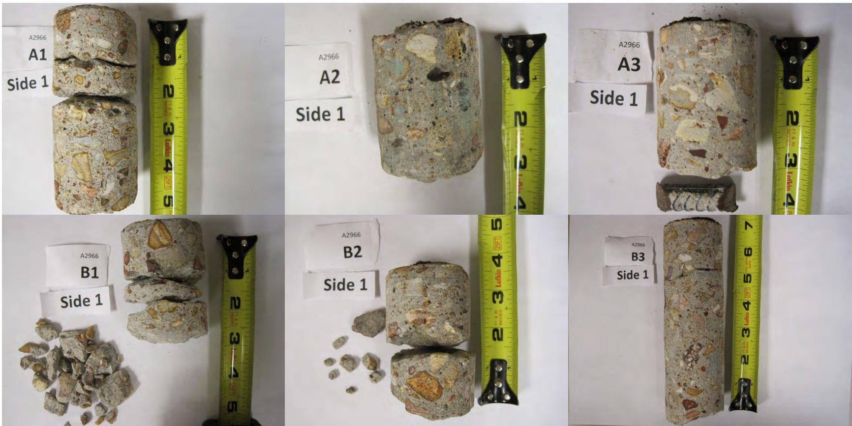
Figure 4-14 Cores Extracted From Bridge A2966
