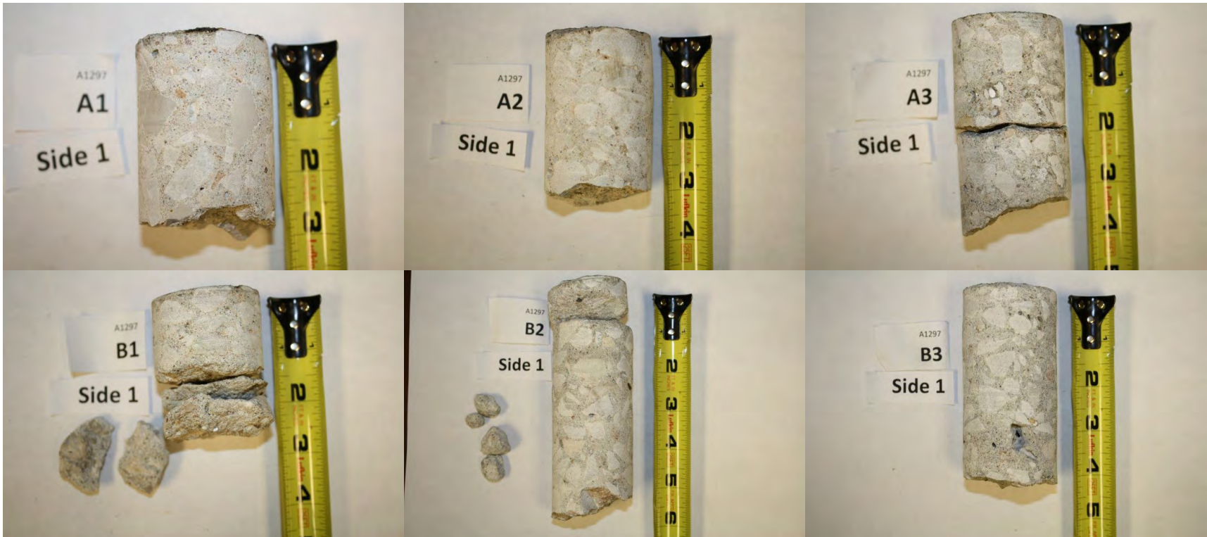
Figure 4-8 Cores Extracted From Bridge A1297
