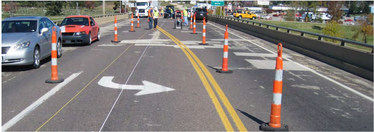
Figure 3-8 Bridge A2966 Overview of Bridge Deck Observed During Field Investigation
