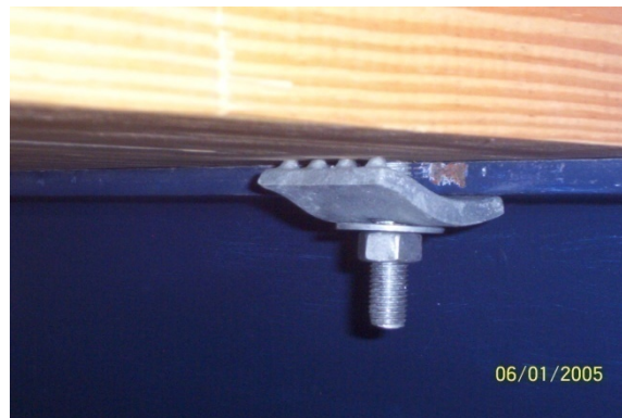
Figure 2. Deck-to-Girder Connection
