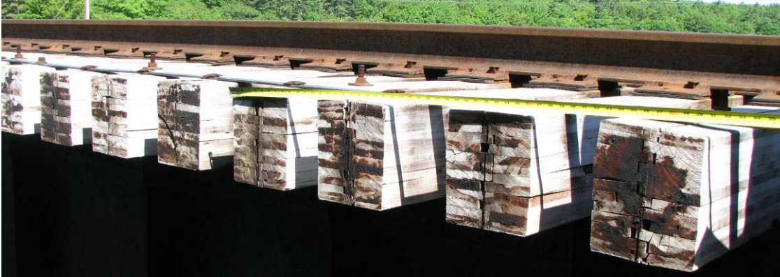
Figure 5: End view of AEL ties
