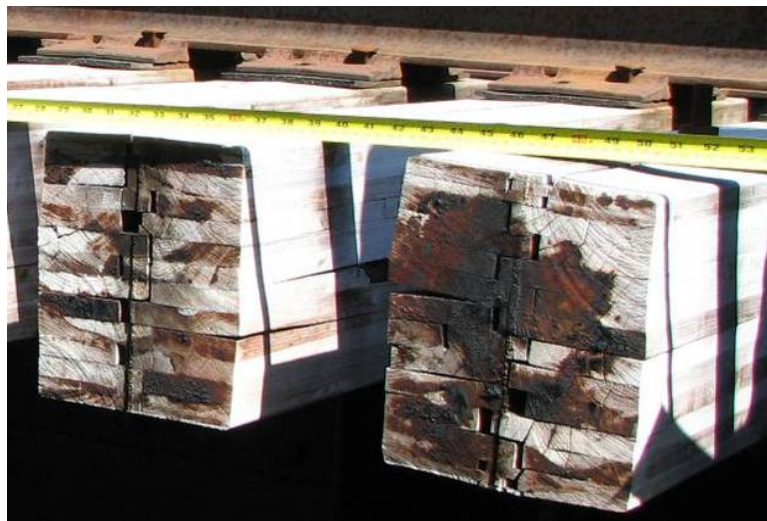
Figure 6: First 2 ties on east end-south overhang
