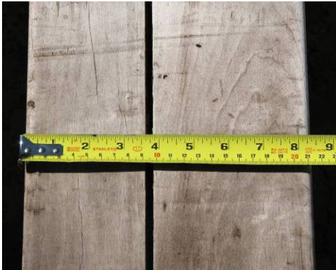
Figure 2: Top view of bridge ties
