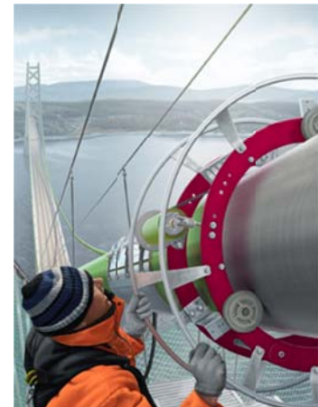
Figure 21: Cableguard™ wrapping application. [dsbrown.com]
