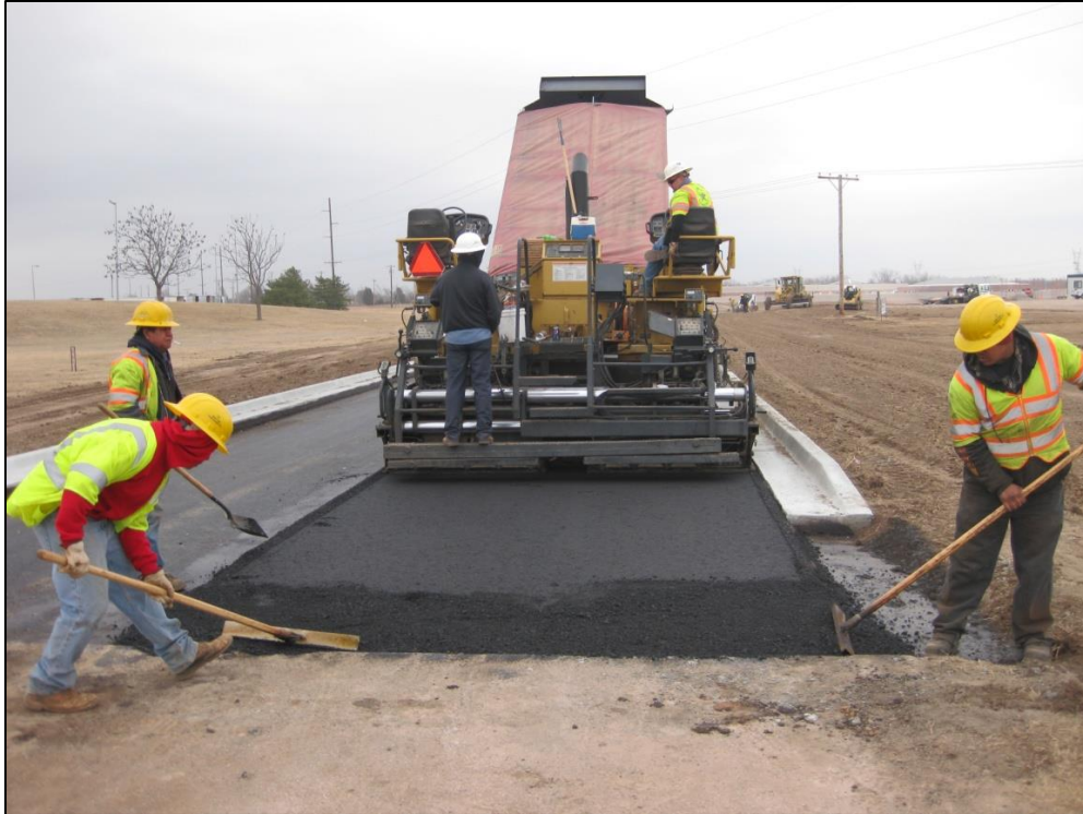
Figure 3.11 Laydown of S4-0 Layer (South Lane).
