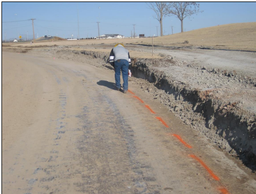
Figure 3.7 Stabilized Subgrade.
