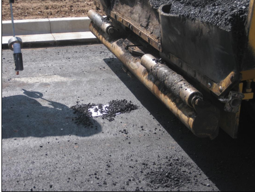
Figure 3.13 Placement of Paper During Laydown of S4 Layers.
