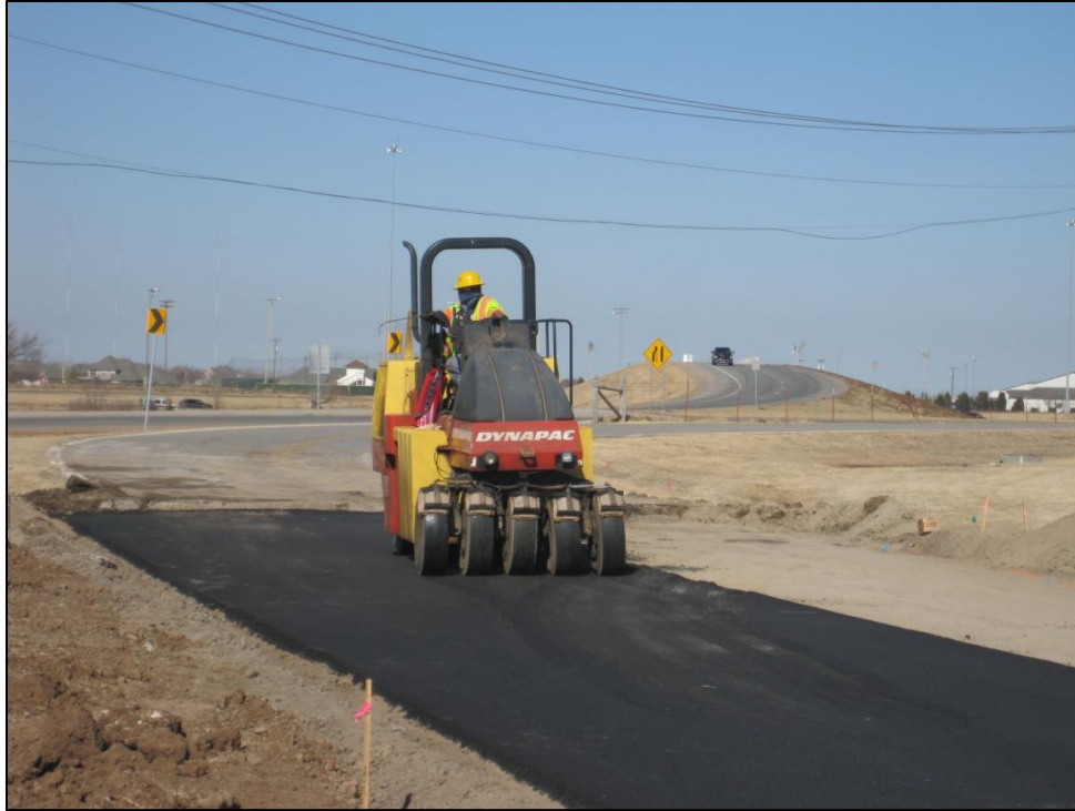
Figure 3.10 Compaction of S3-25 Layer With Rubber-Tire Roller.
