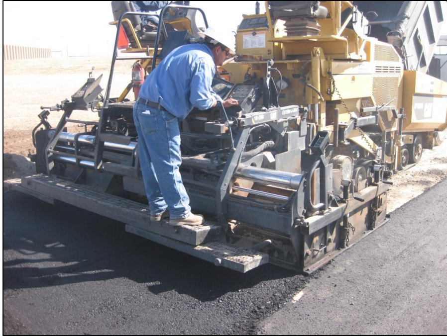
Figure 3.14 Laydown of S3-40 Layer (North Lane).
