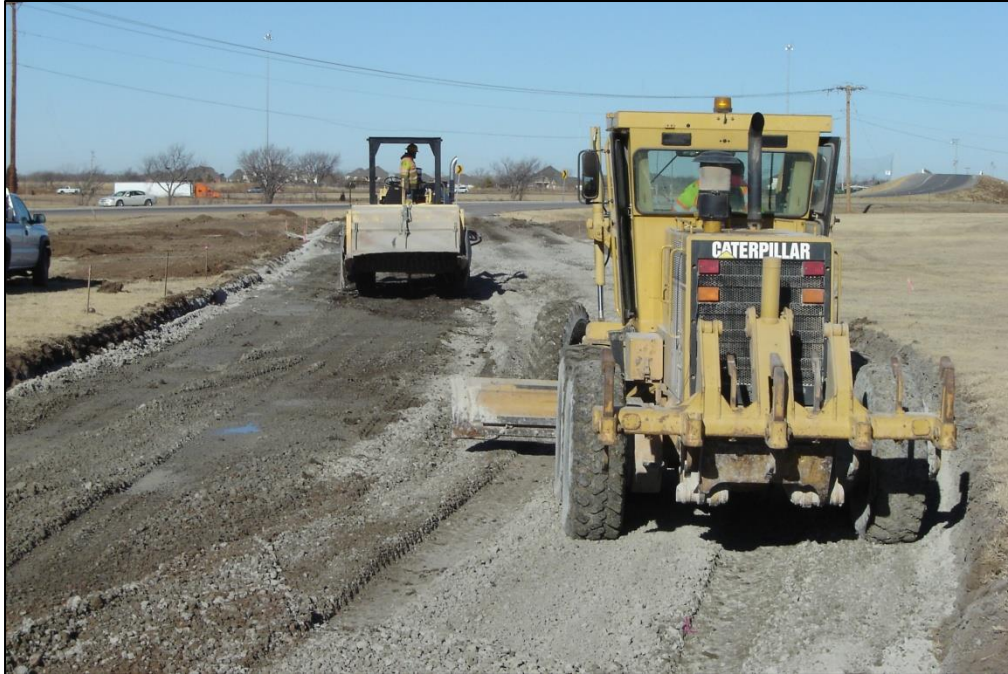
Figure 3.4 Process of Mixing CKD With the Subgrade.
