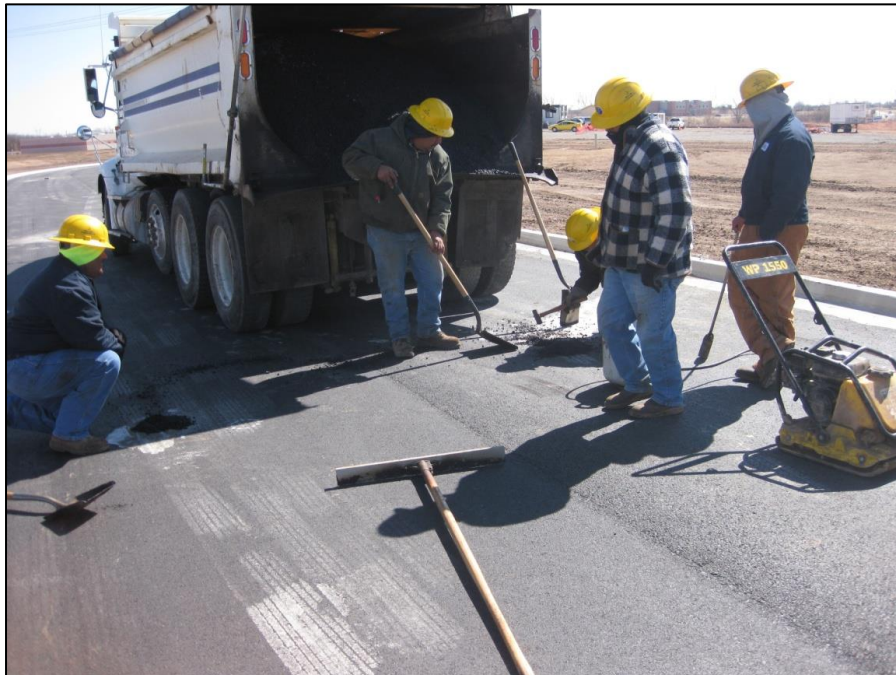
Figure 3.18 Patching Process of the Holes.
