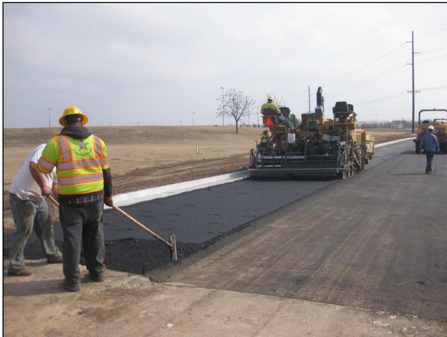
Figure 3.15 Laydown of S4-10 Layer Over S3-40 Layer (North Lane).
