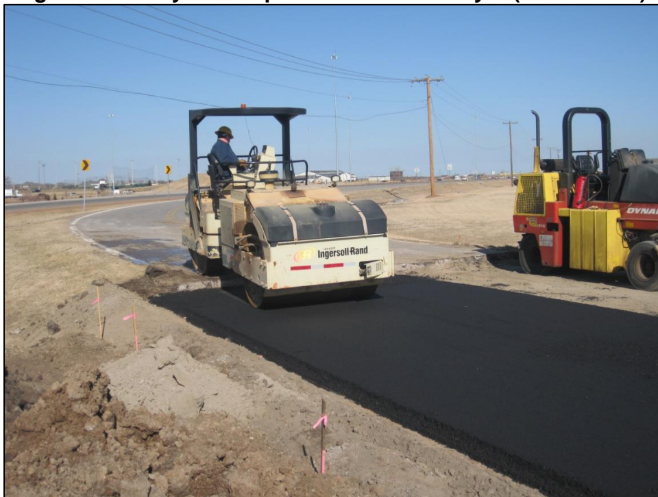
Figure 3.9 Compaction of S3-25 Layer with Steel Drum Roller
