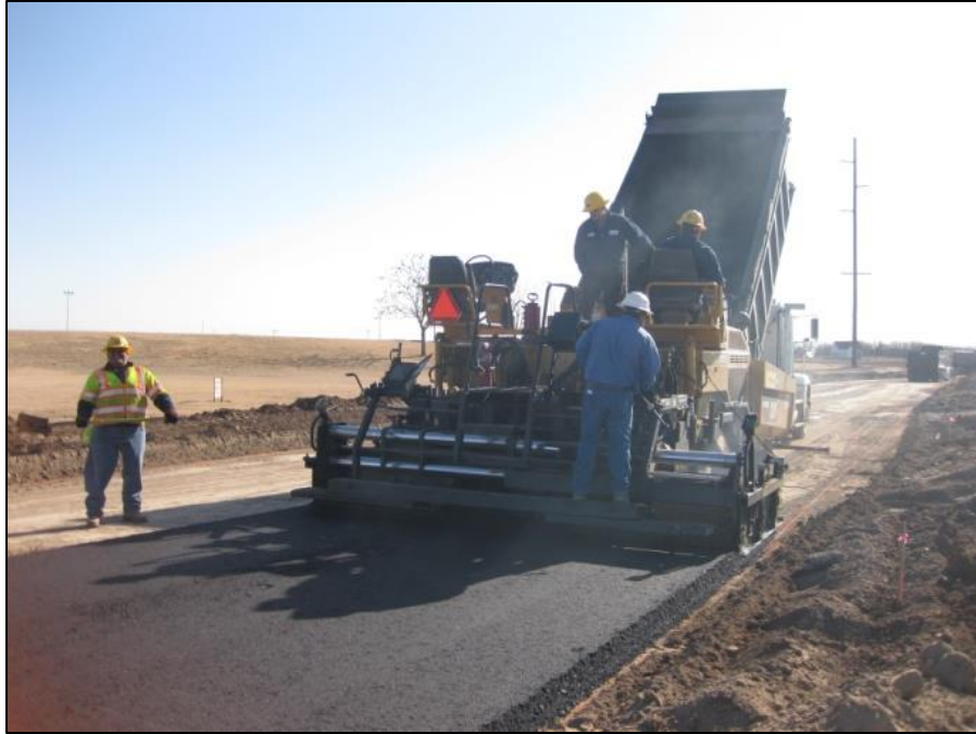
Figure 3.8 Laydown Operation of S3-25 Layer (South Lane).
