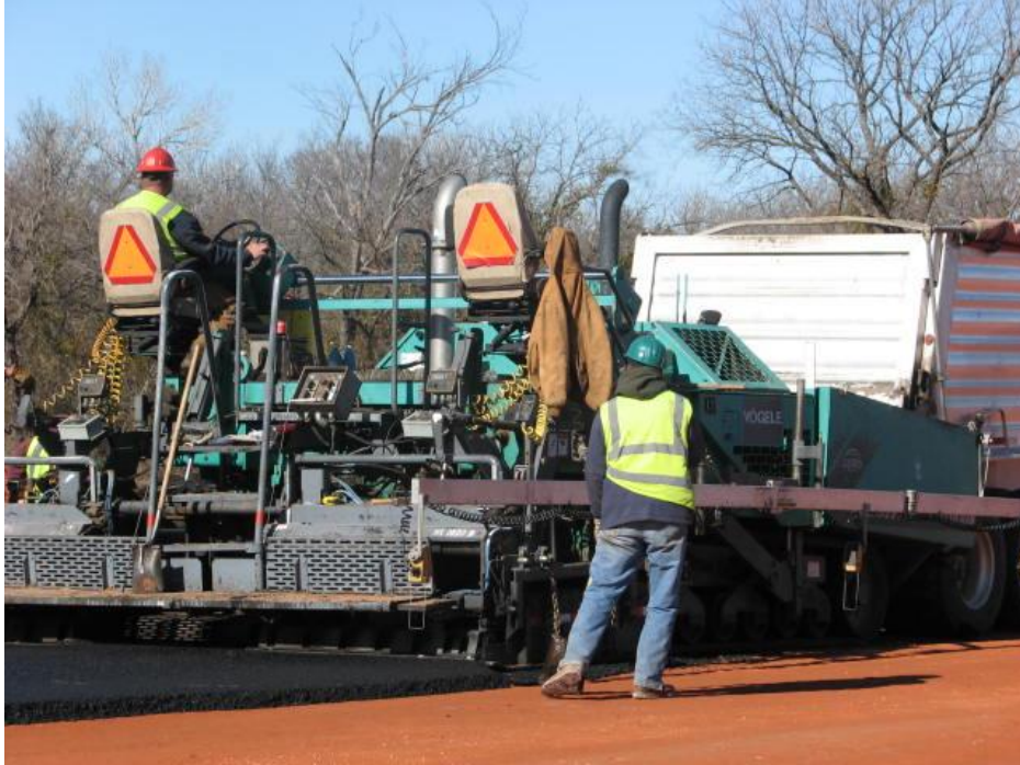
Figure 3.21 The Paving Machine Used for Test Site 2.
