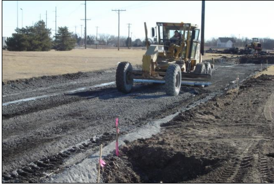
Figure 3.6 Leveling of the Stabilized Soil.
