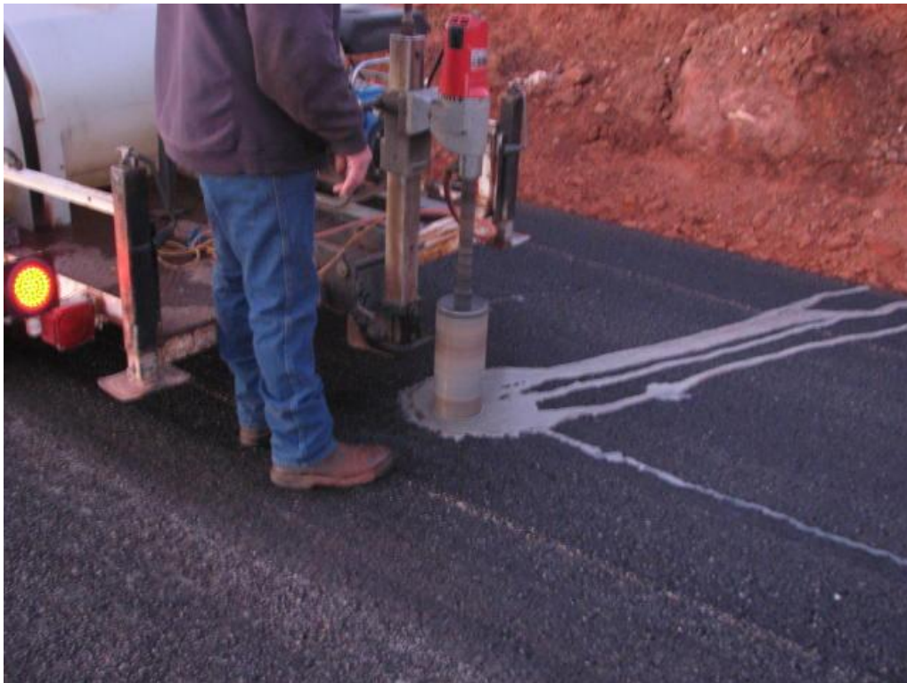
Figure 3.24 Coring in Progress for Test Site 2.
