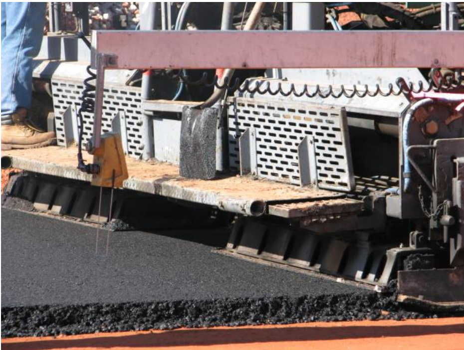
Figure 3.22 Construction of S3 Lift for Test Site 2.
