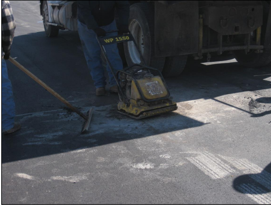
Figure 3.19 Plate Compaction During Patching Holes.
