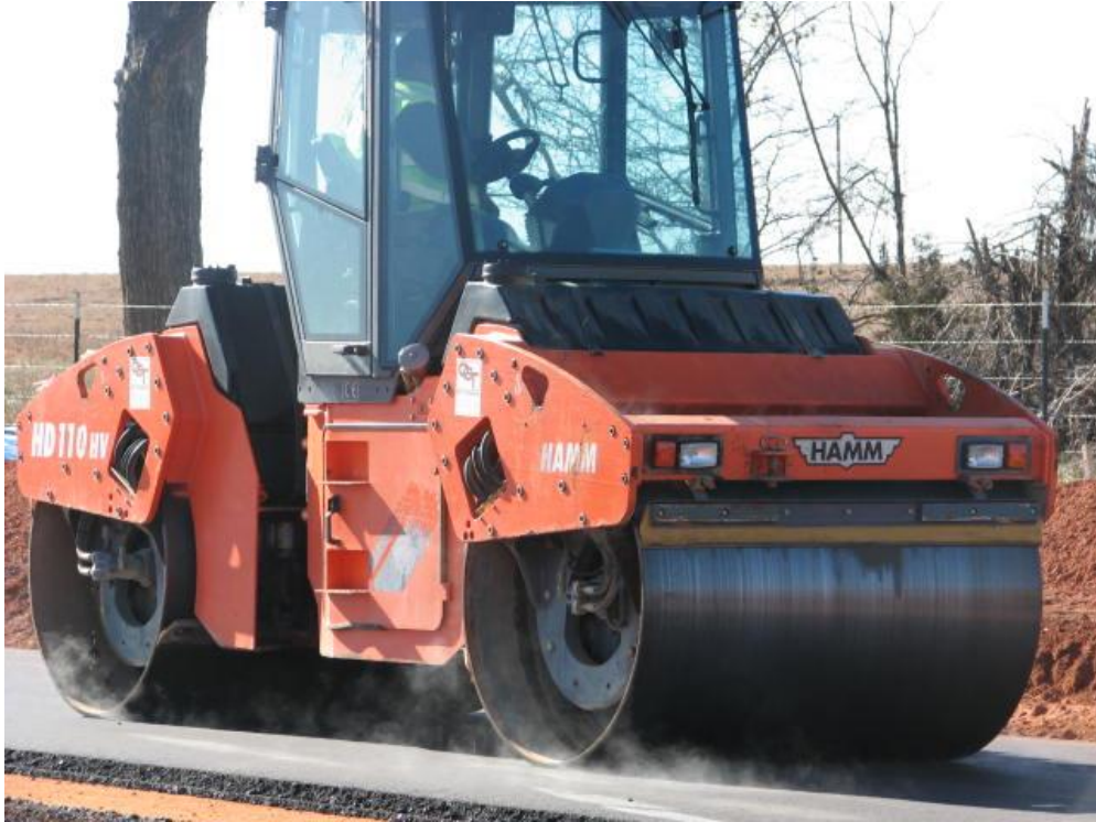
Figure 3.23 Compaction of S3 Lift for Site 2.
