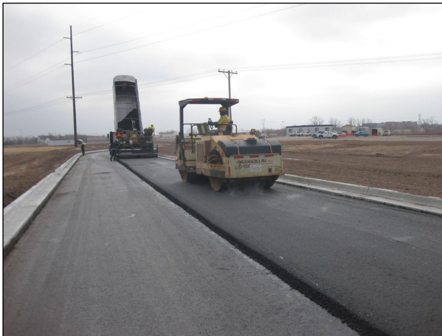
Figure 3.12 Laydown and Compaction of S4-0 Layer (South Lane).
