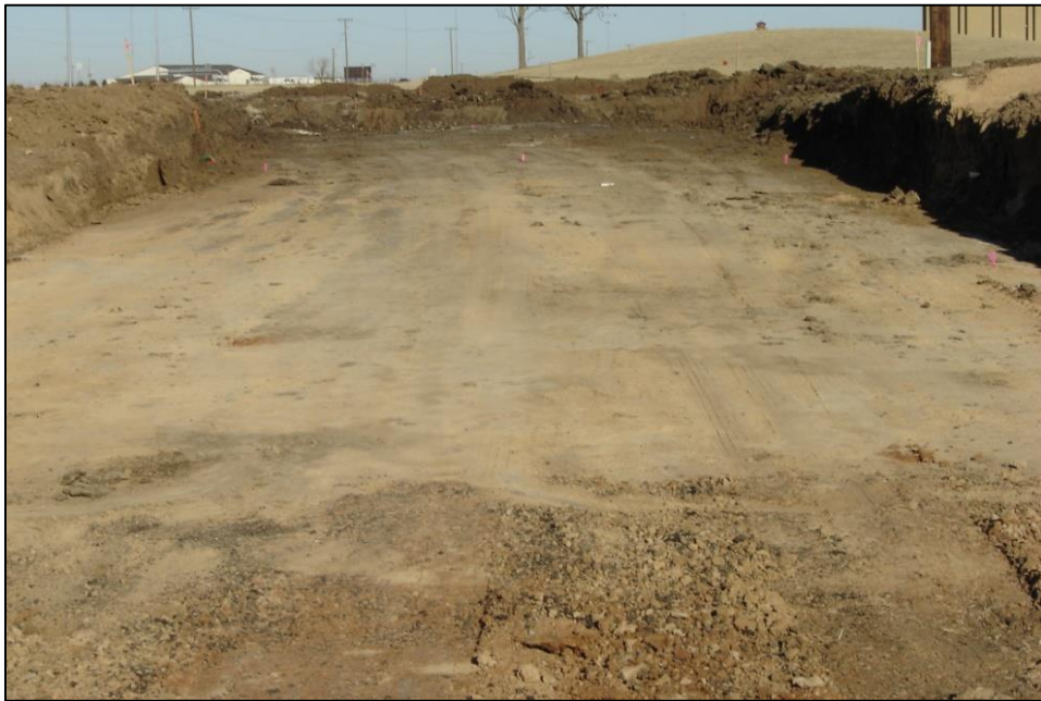
Figure 3.3 Right of Way Before Soil Stabilization.
