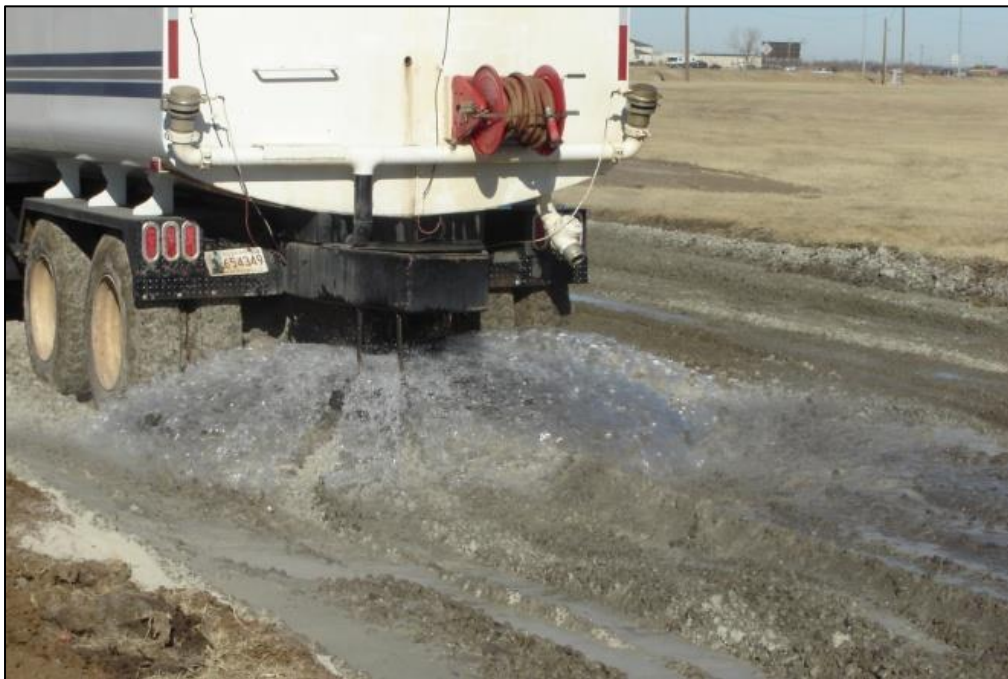
Figure 3.5 Watering During the Stabilization Process.
