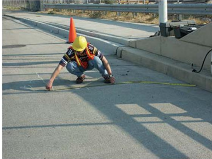
Figure 1.2 A human inspector measures cracks for bridge deck maintenance.
