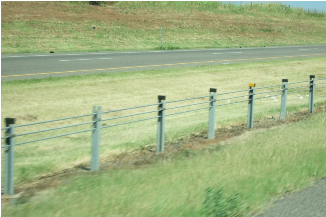
Figure 19 CASS 3 cable system on C-Shaped posts
