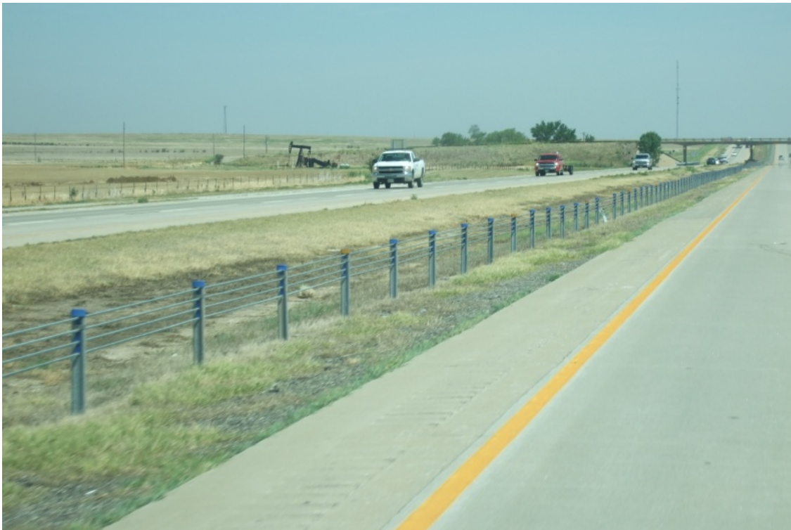
Figure 26 Cable Barrier Located Between Center and Edge of Median
