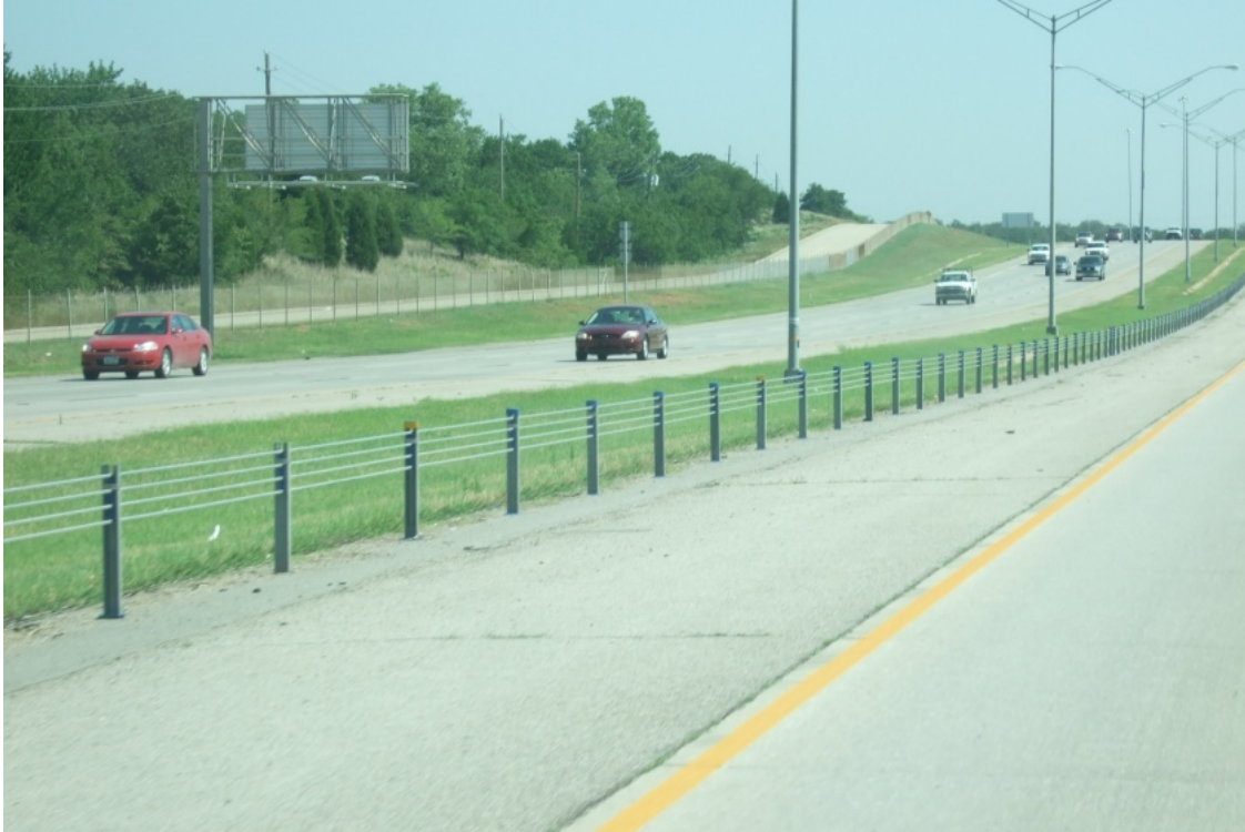
Figure 25 Cable Barrier Along Interior Shoulder
