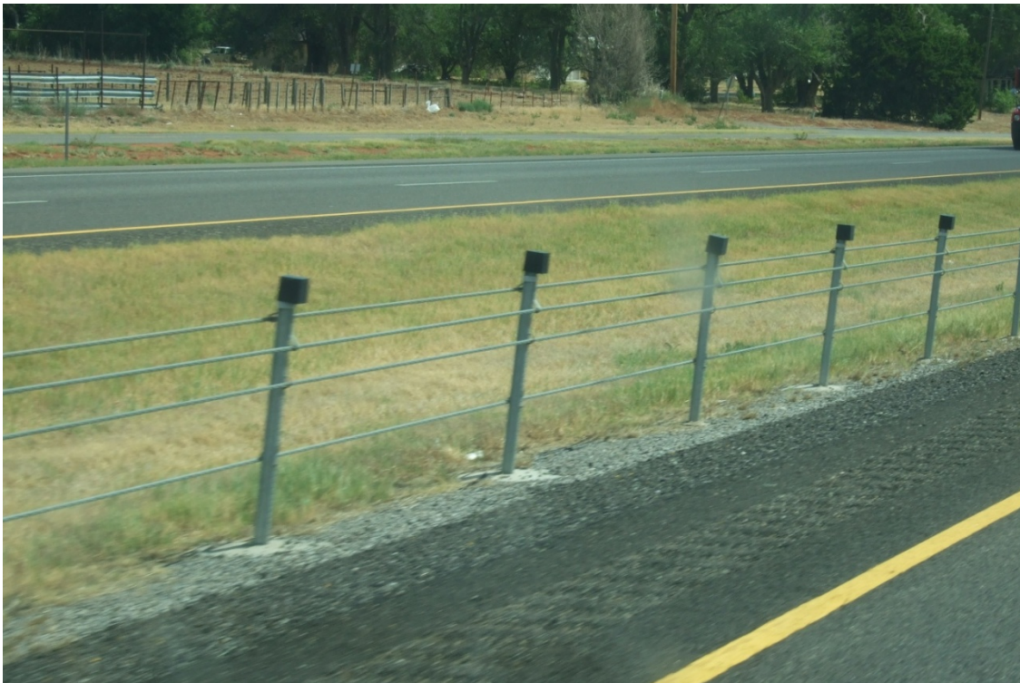
Figure 21 U.S. High-Tension Cable System by Nucor Steel Marion Inc.
