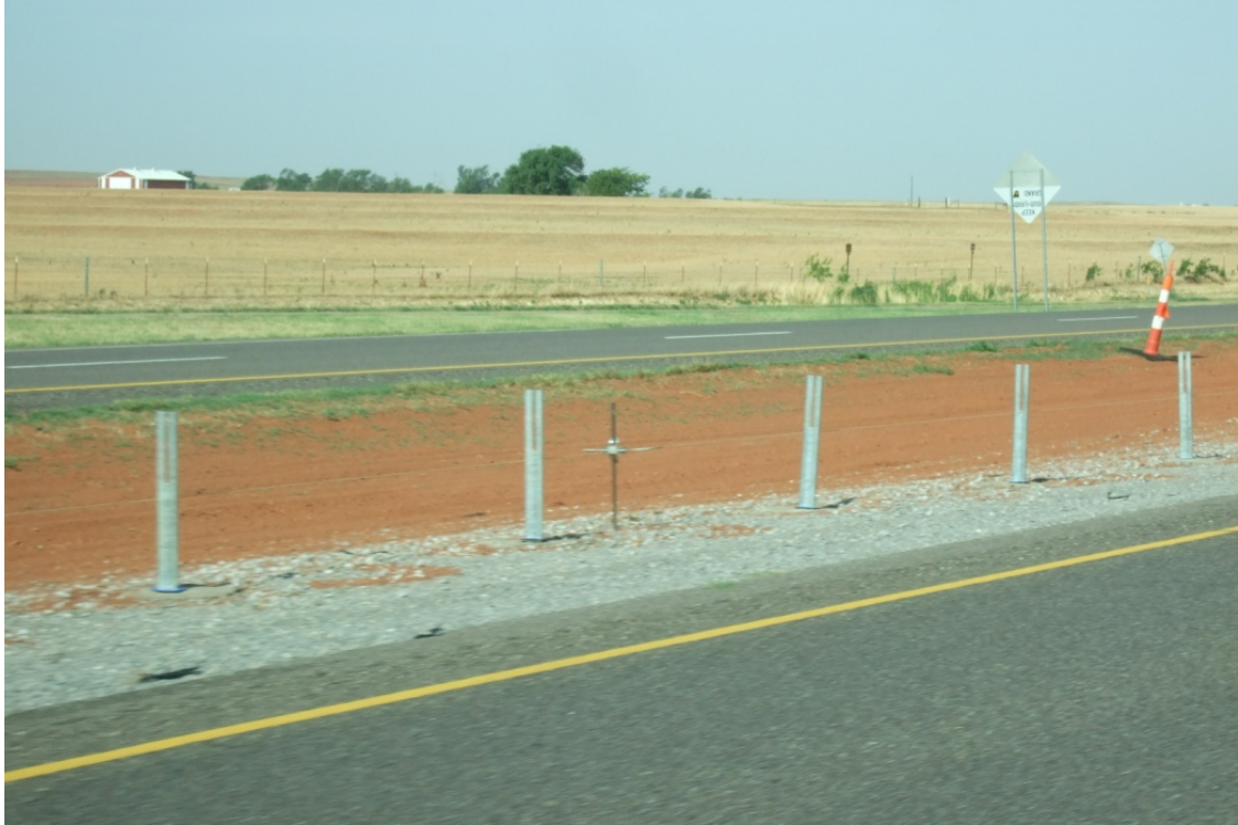
Figure 6 Cable Barrier Installation on I-40
