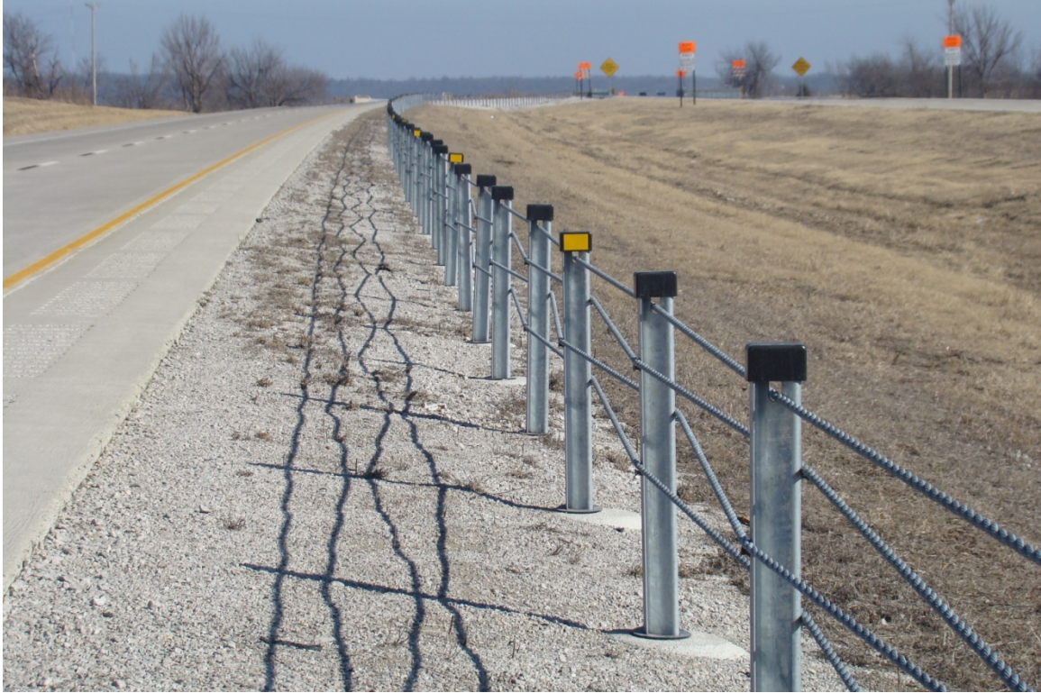
Figure 13 Cable Barrier installed at median edge
