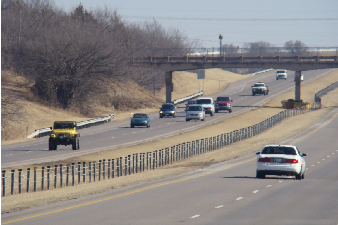
Figure 11 Cable Barrier on I-40
