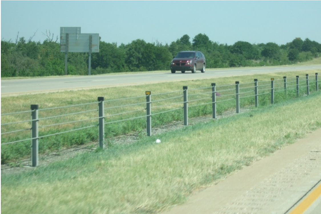
Figure 24 Cable Barrier in Center of Median
