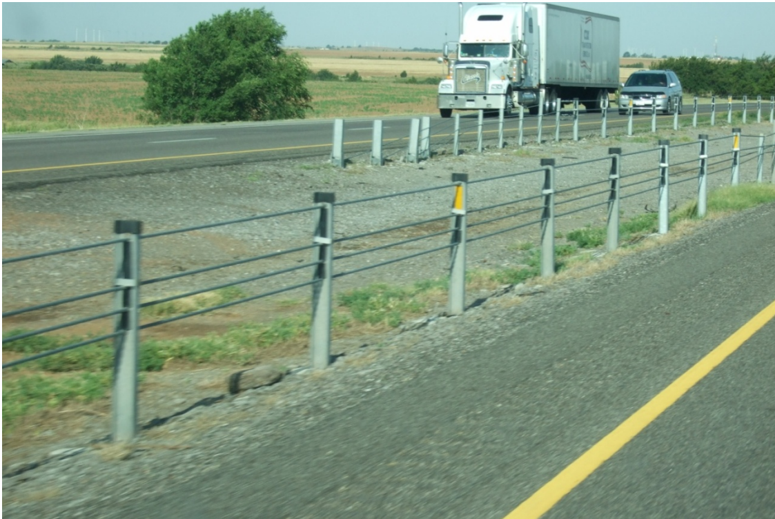
Figure 20 Trinity CASS 4 Barrier with 4 cables
