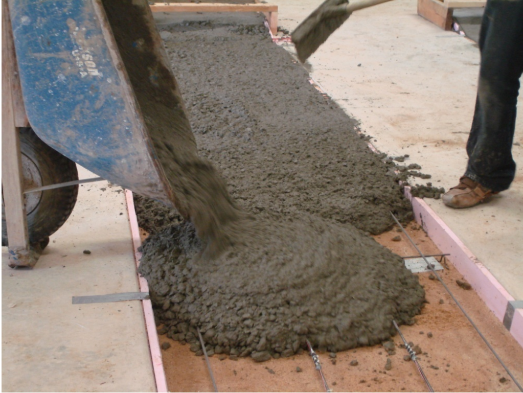
Figure 4.14: Casting Slab
