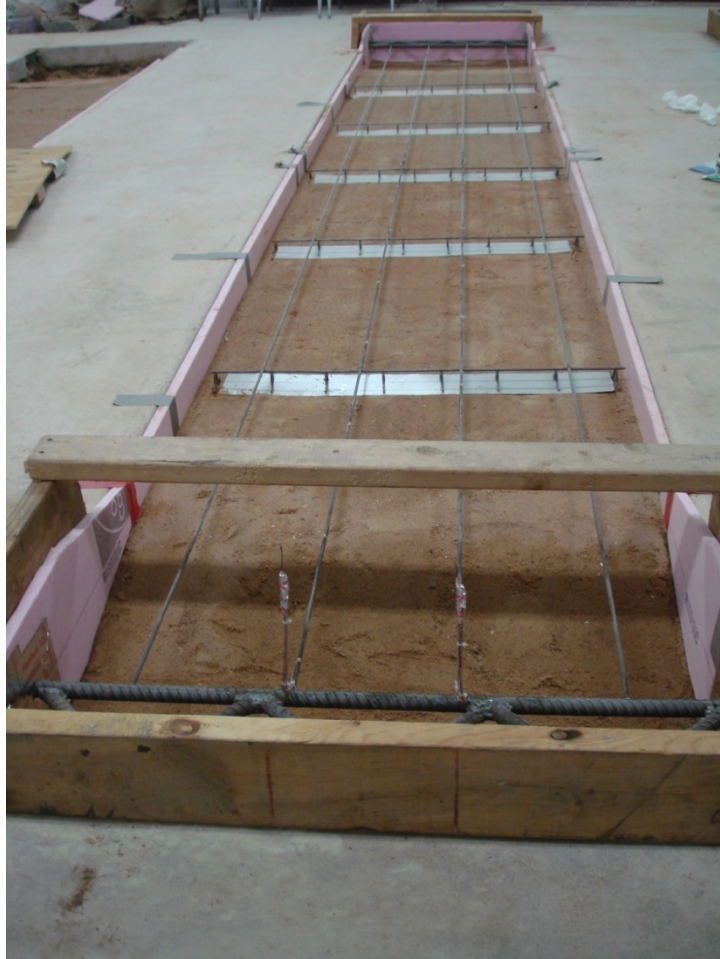
Figure 4.11: Slab is ready to be cast
