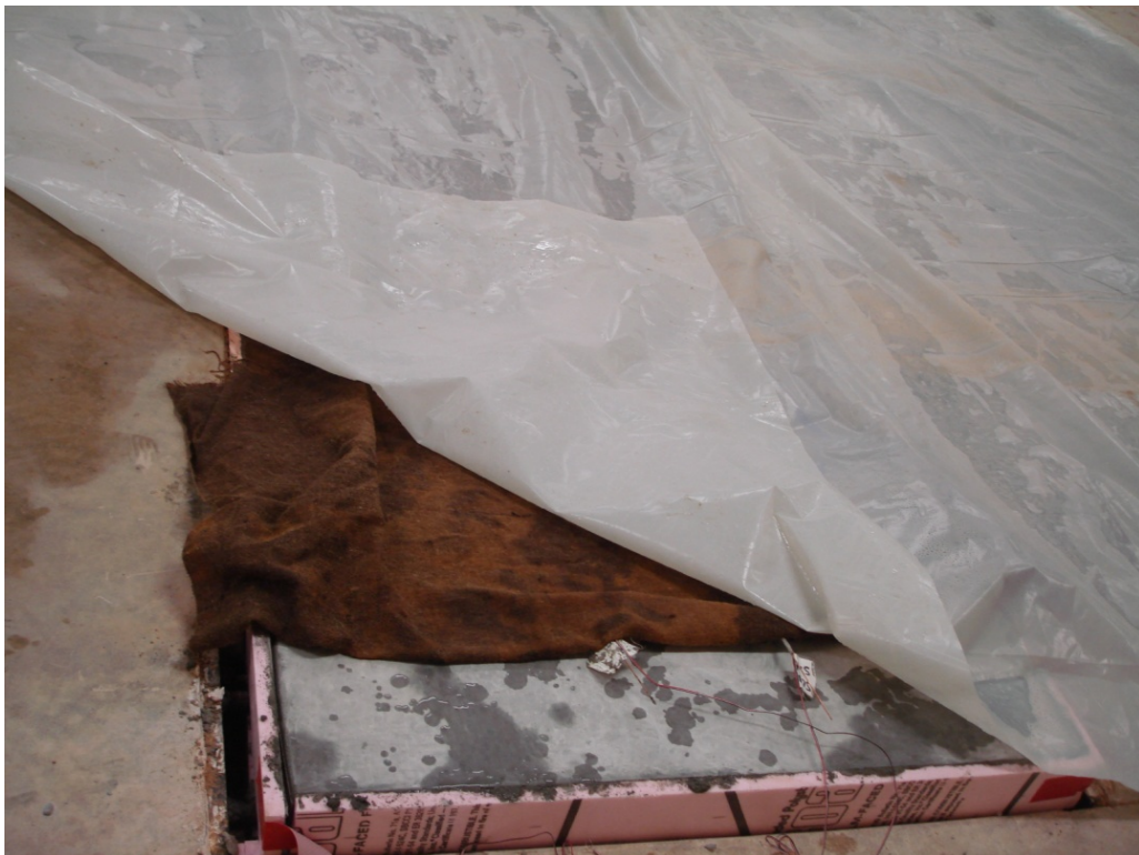
Figure 4.19: Curing Concrete with Wet Burlap Covered by Plastic Sheet
