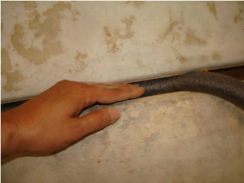
Figure 4.39: Placing Backer Rod in the Gap at the Slab Edge
