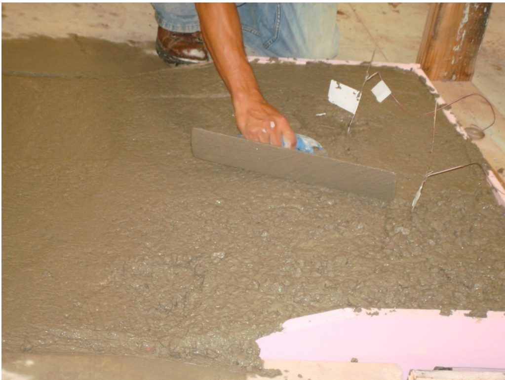
Figure 4.15: Finishing Concrete Surface (End of the Slab)
