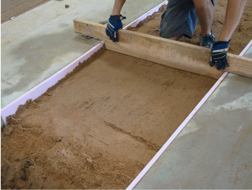
Figure 4.7: Compacting Sand
