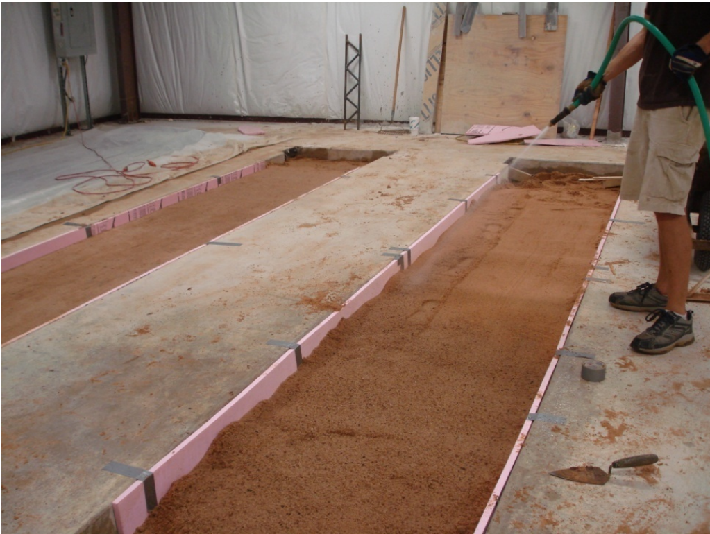
Figure 4.5: Watering Sand to help compact the sub-base
