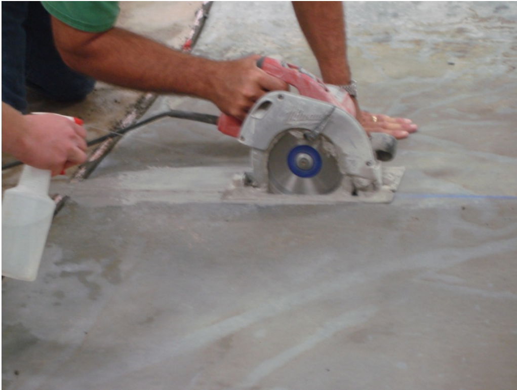
Figure 4.20: One inch Depth Joint Using Saw Cut
