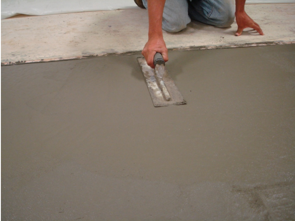
Figure 4.16: Finishing Concrete
