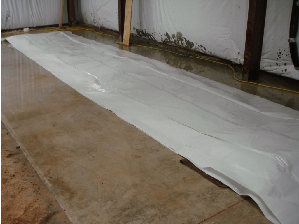
Figure 4.18: Moist Curing of Slabs
