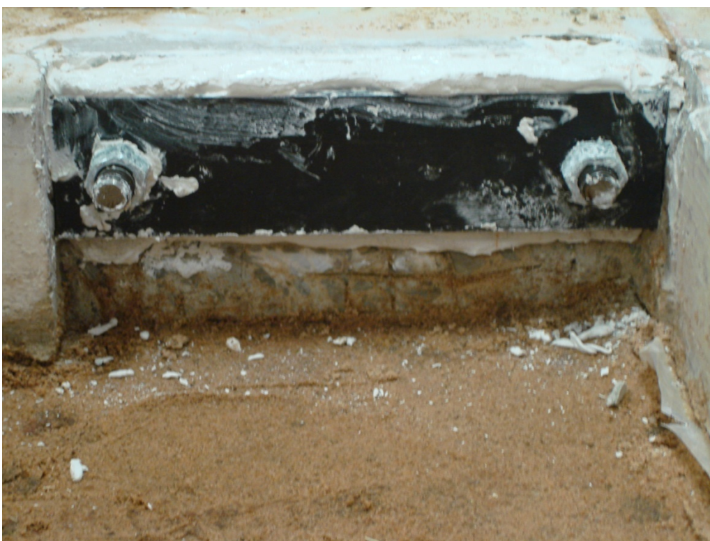
Figure 4.3: Using Grout between Plate and Existing Slab
