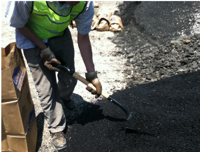
Figure 3.6 Advera ® WMA Mix Collection from Asphalt Plant in Bridgeport, TX
