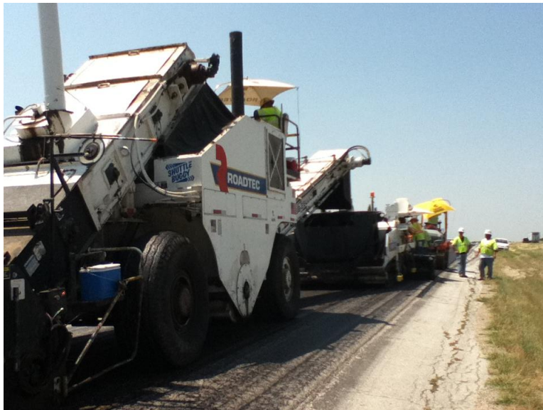
Figure 3.8 Overlay Project in US 287 using Advera ® WMA
