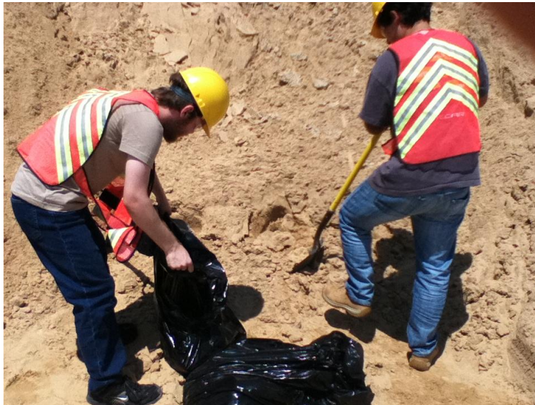
Figure 3.4 Collection of Natural Sand from the Asphalt Plant in Bridgeport, TX
