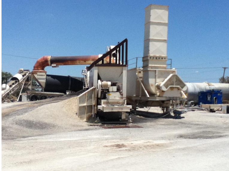
Figure 3.1 Photographic View of the Asphalt Plant in Bridgeport, TX
