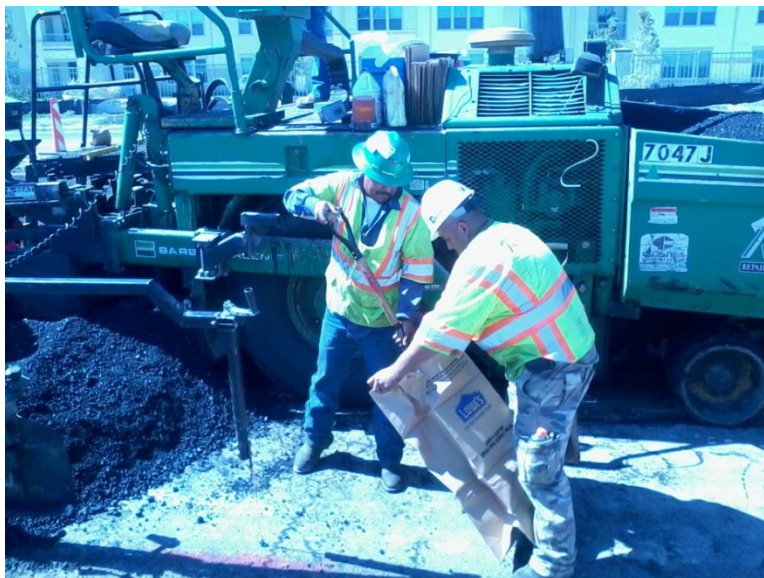
Figure 3.10 Evotherm ® Type B Mix Collection from Foster Road, San Antonio, TX
