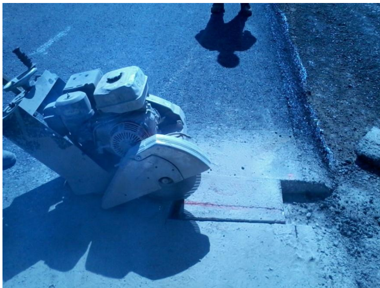
Figure 3.14 Cutting of Slab Samples
