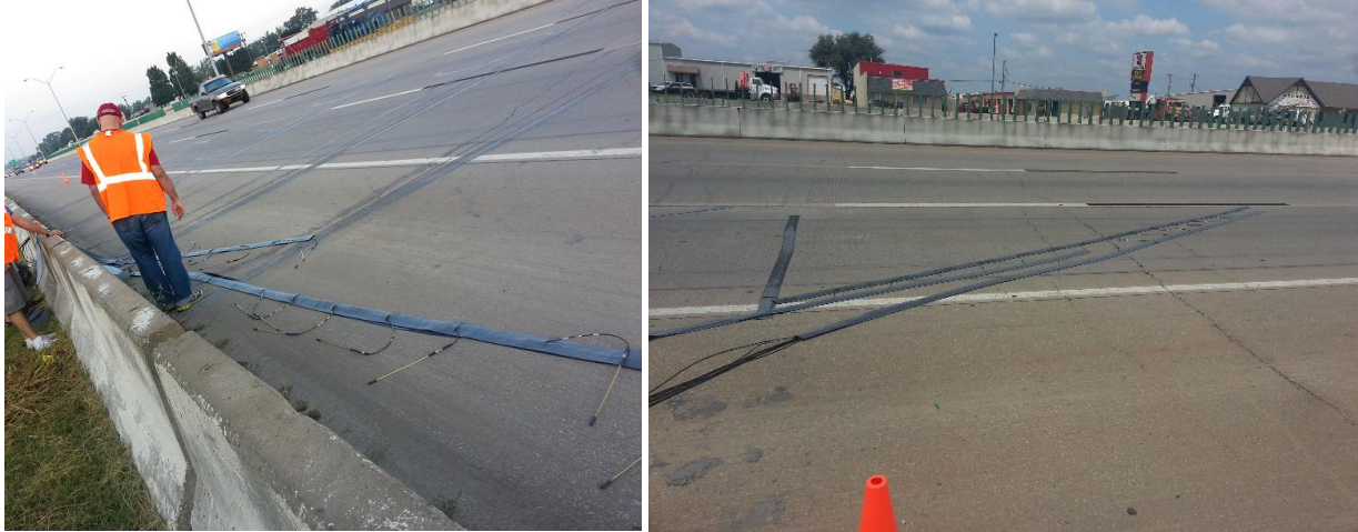
Figure 6.3. AVC19 deployment site and sensor layout
