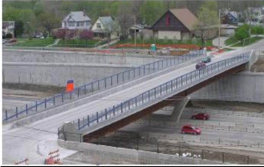
Figure 2.1 The East 12 th street Bridge, Des Moines, Iowa
