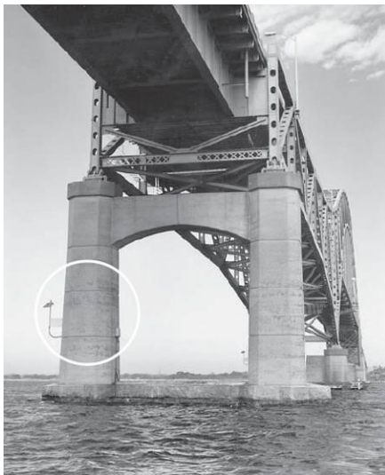
Figure 2.2. Scour monitoring system mounted on a pier on the Robert Moses Causeway over Fire Island Inlet, New York (circled) (Copyright: Raimondo di Egidio 2002, cited by Hunter 2009).
