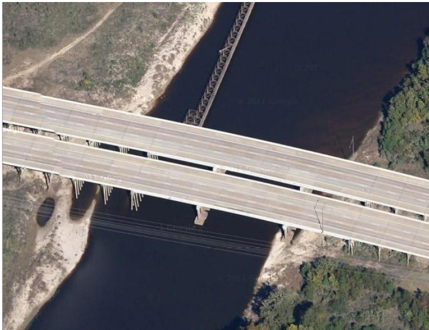
Figure5.1 SR 25 Bridge #1.7A on Lakeland Drive over the Pearl River in Jackson, Mississippi
