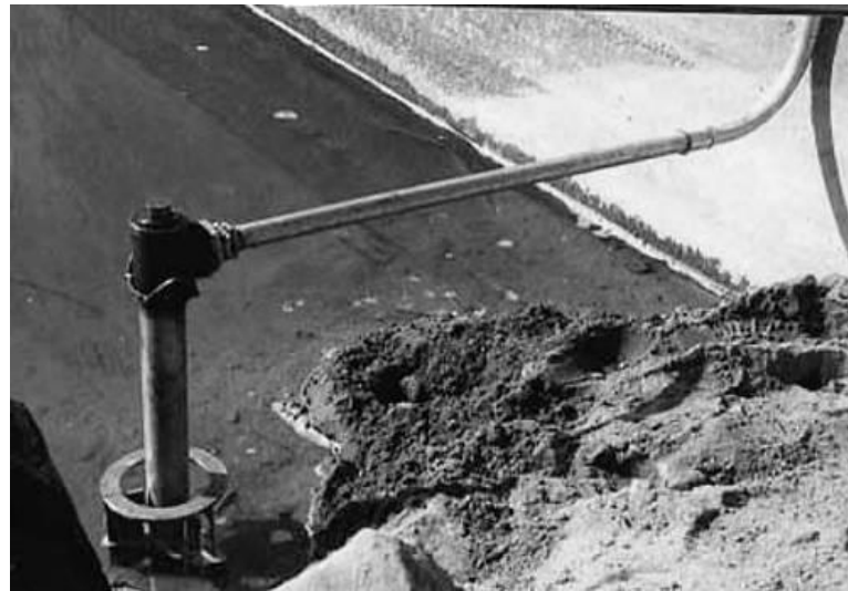
Figure 2.7. Magnetic sliding collar installation (Hunter 2009)
