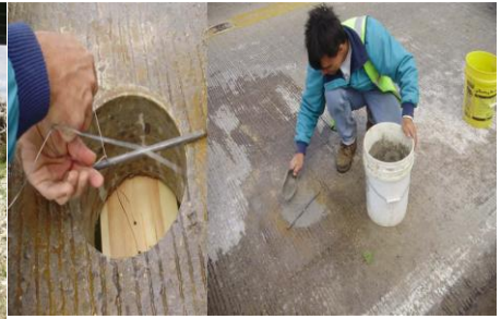
Figure 4.8 Finishing of installation (courtesy of Bill Yu)
