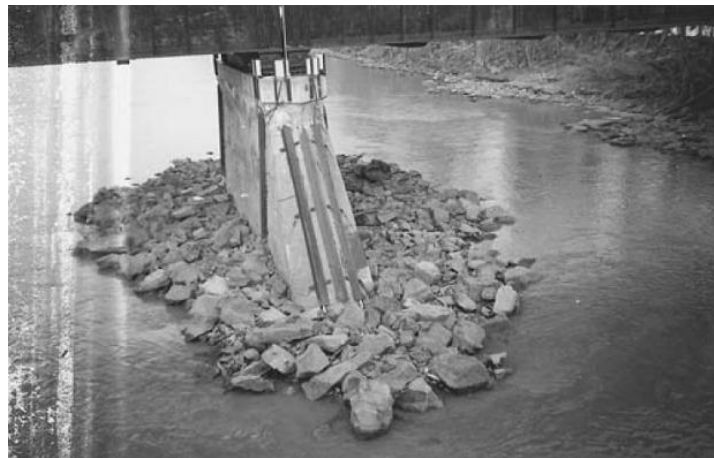
Figure 2.13. Sounding rods installed to monitor riprap in New York (Hunter 2009).
