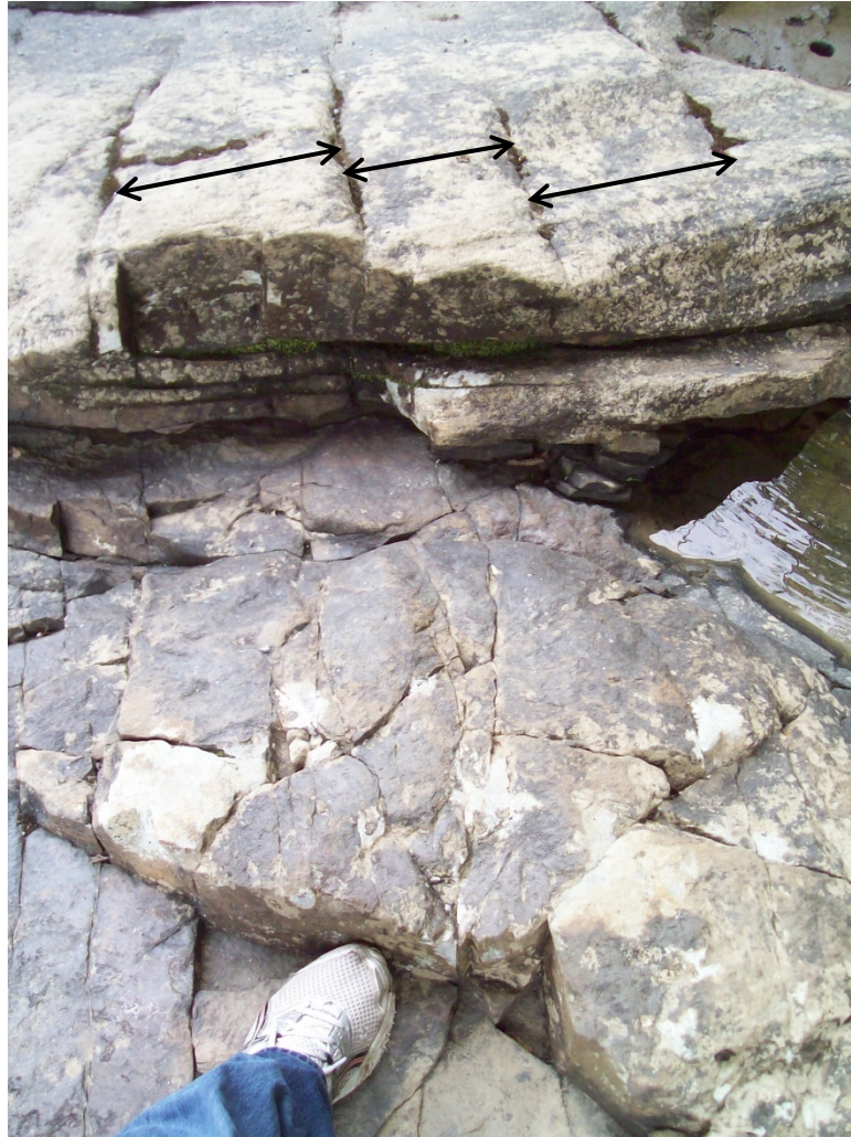
Figure 11 – Example of jointing (Audra Park Bridge). Arrows show joint spacing
