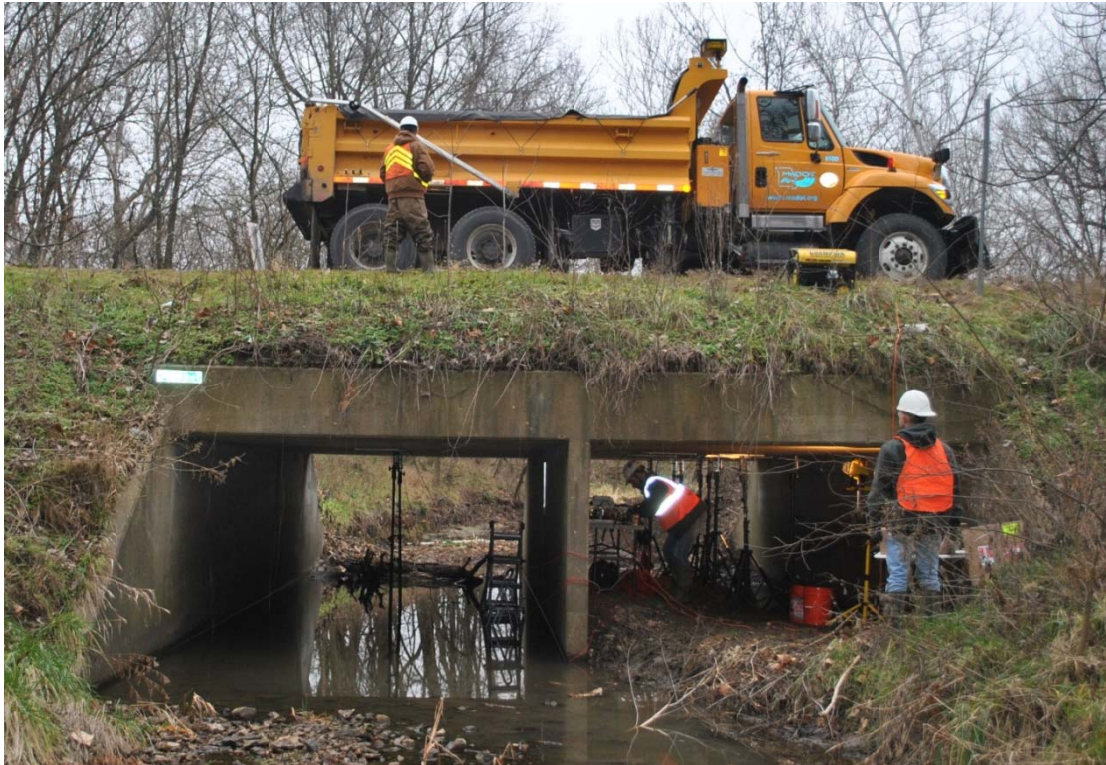
Figure 3-5 – Photograph of testing with truck in Position 2.
