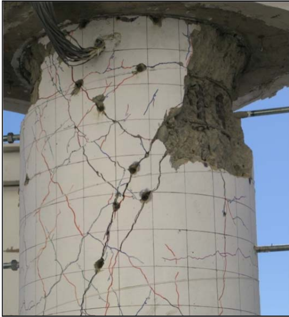
Damage state of as-built specimen SP1
