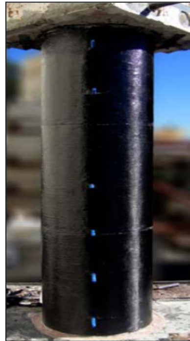
CFRP repaired SP2
