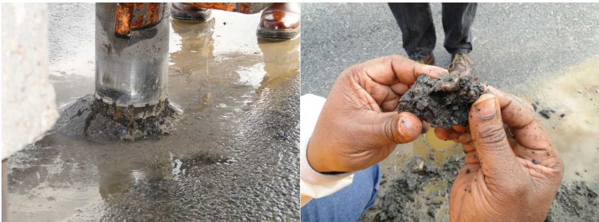
Figure 6 Observation of moisture damage during coring
