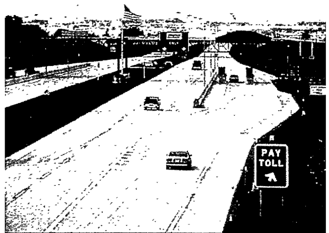
Oklahoma City saved $160,000 per year per toll booth when booths were equipped with electronic debit systems.
