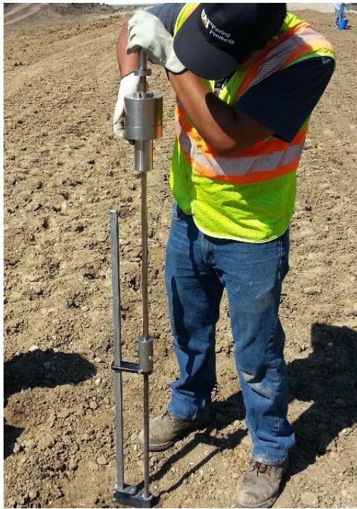
Figure 29. Dynamic cone penetrometer testing
