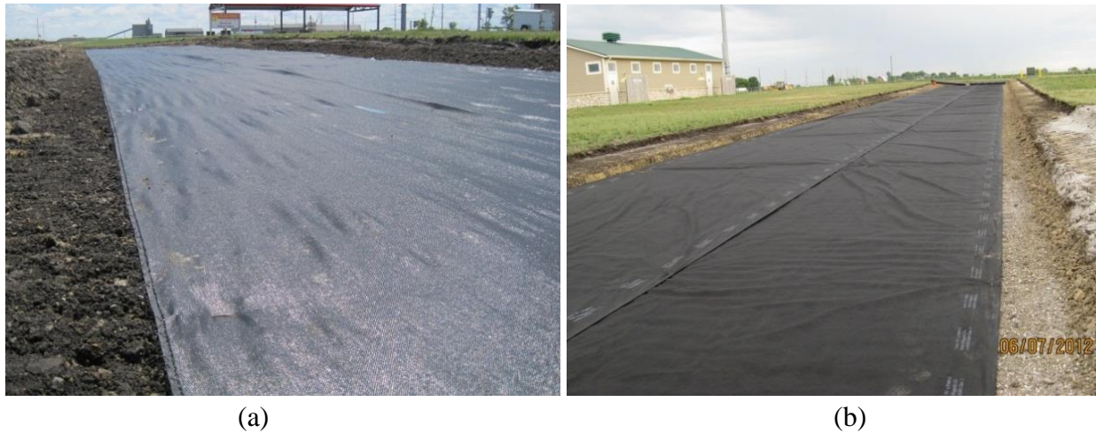
Figure 19. Geotextiles placed at subgrade/aggregate layer interface: (a) woven geotextile, and (b) non-woven geotextile (pictures from Boone County Expo Site, June 2012)
