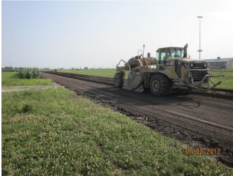
Figure 16. Blending granular material with subgrade using a soil pulverizer (picture from Boone County Expo Site, June 2012)
