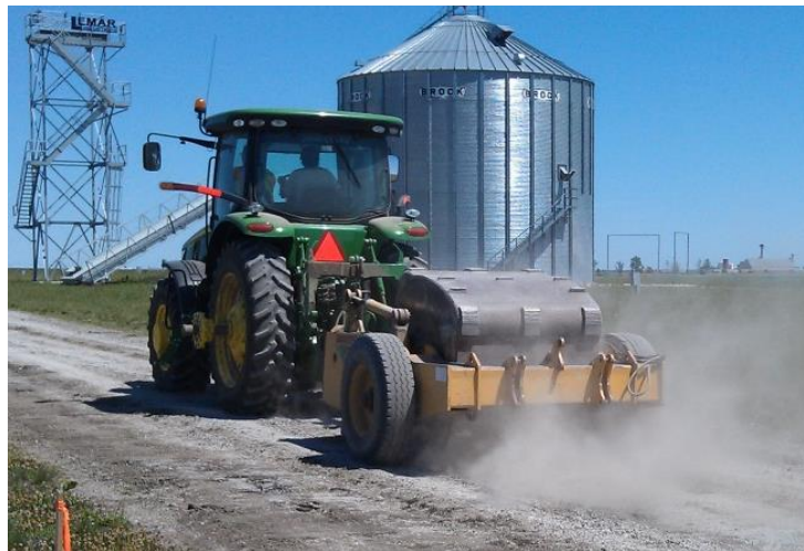
Figure 18. High energy impact roller equipment by equipment by Impact Roller Technology, Plattsmouth, Nebraska (picture from Boone County Expo Site, June 2012)
