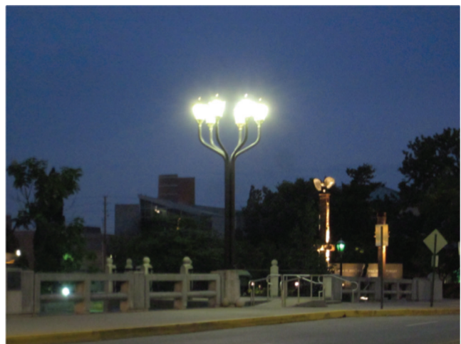
Figure 2.5 Induction lighting on Ohio Street.
