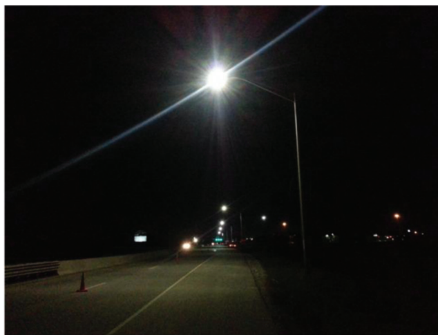
Figure 2.2 MH lighting on US-231.
