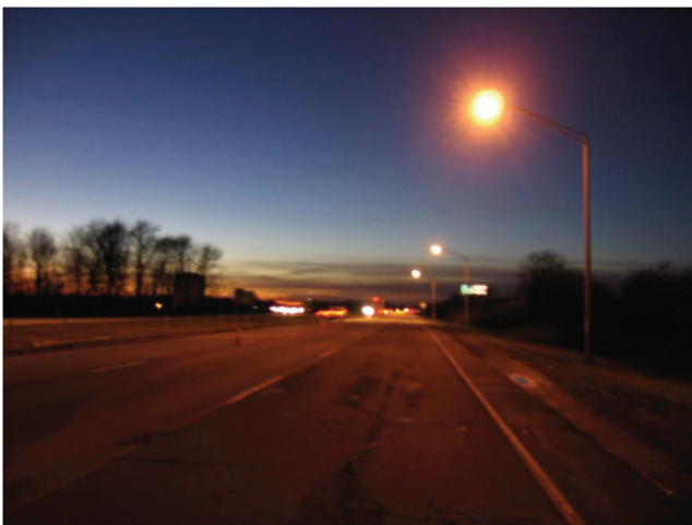
Figure 2.1 HPS lighting at I-74/US-231 interchange.
