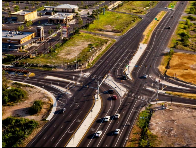
Figure 3.4. Aerial view of a superstreet in Texas (33).
