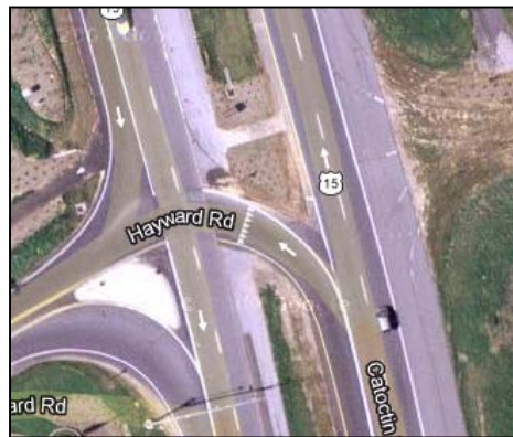
Figure 3.3. Pedestrian crossing through the median of a J-turn in Maryland (26).
