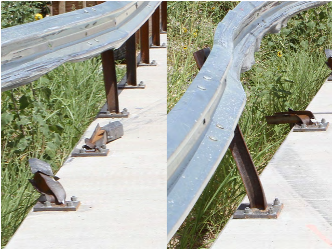
Figure 5.4. Installation after Test No. 490023-6-1a.
