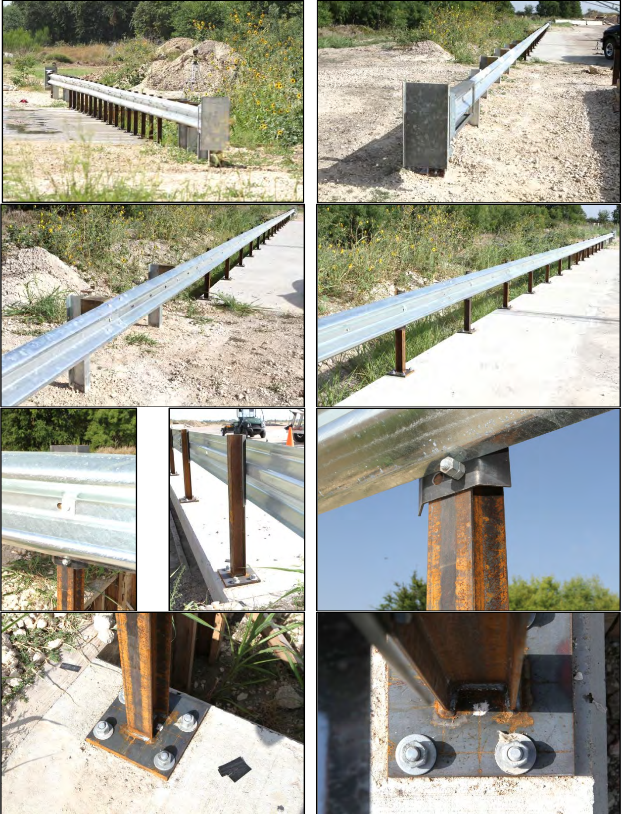
Figure 2.2. T631 Bridge Rail Installation before Test No. 490023-6-1a.
