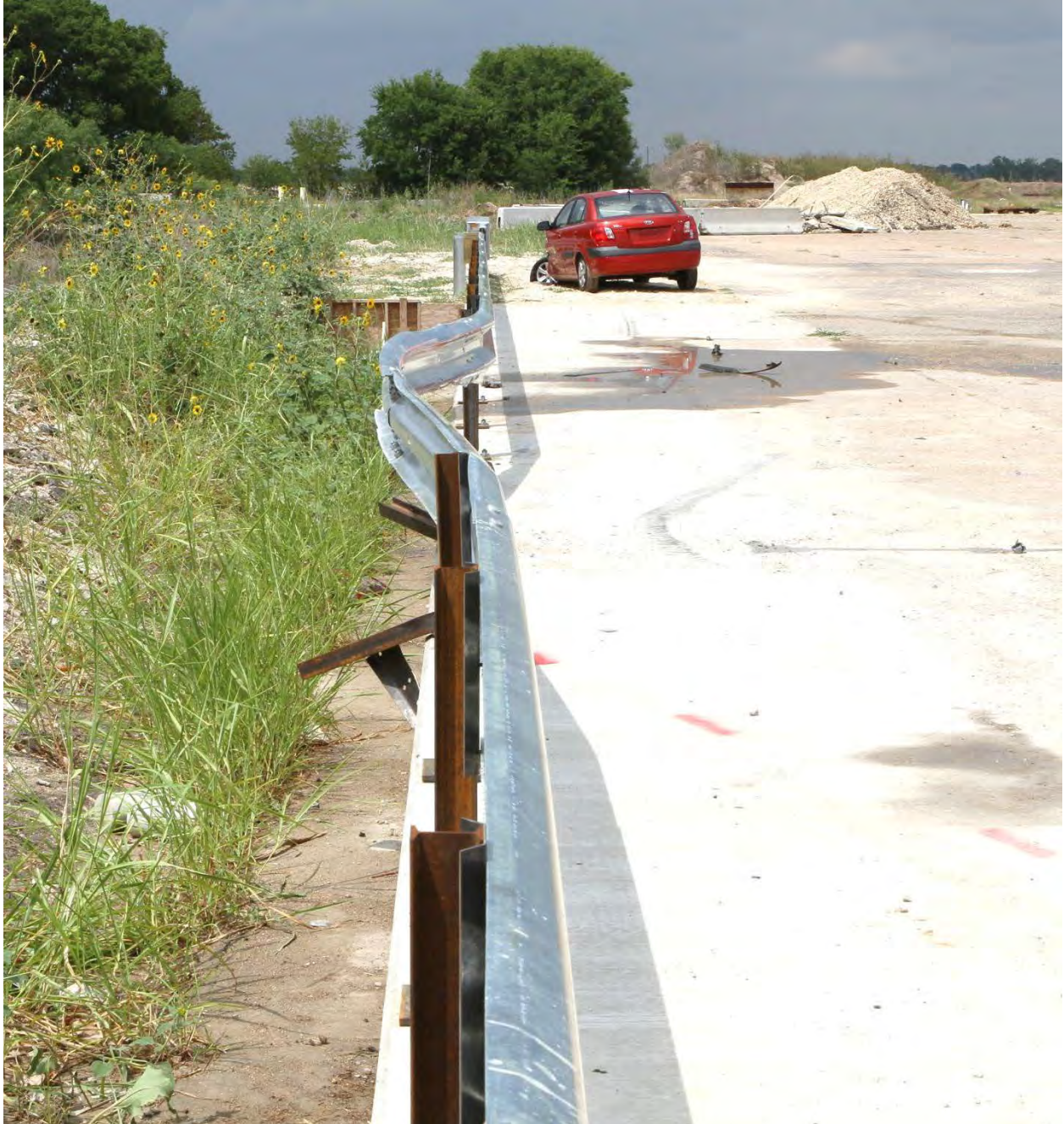
Figure 6.3. Test Article/Vehicle Positions after Test No. 490023-6-2.
