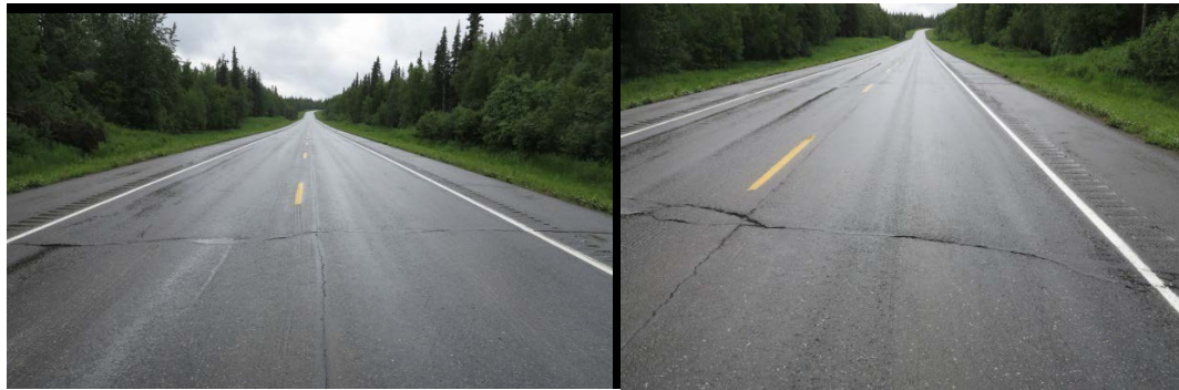
Figure V.15 Severe major transverse cracks with little influence on pavement performance beyond crack edges (very common)
