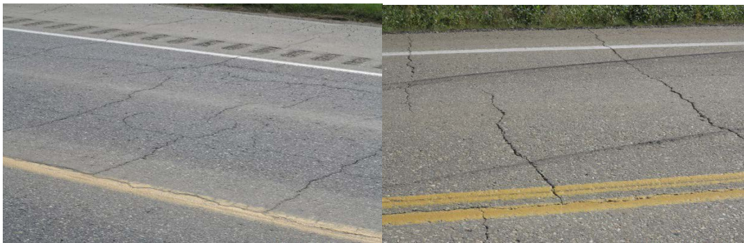
Figure V.14 Lesser thermal cracks showing same performance in wheel path and non-wheel path locations (extremely common appearance)
