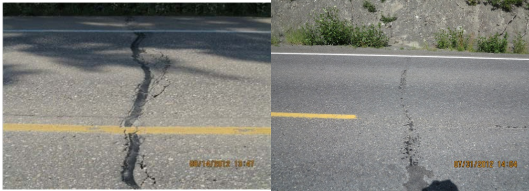
Figure III.2 Major transverse thermal cracks with new sealant (left) and old sealant (right)
