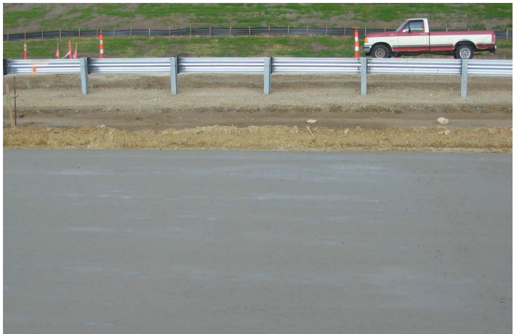
Bleed Water Rising to Surface After Tining
