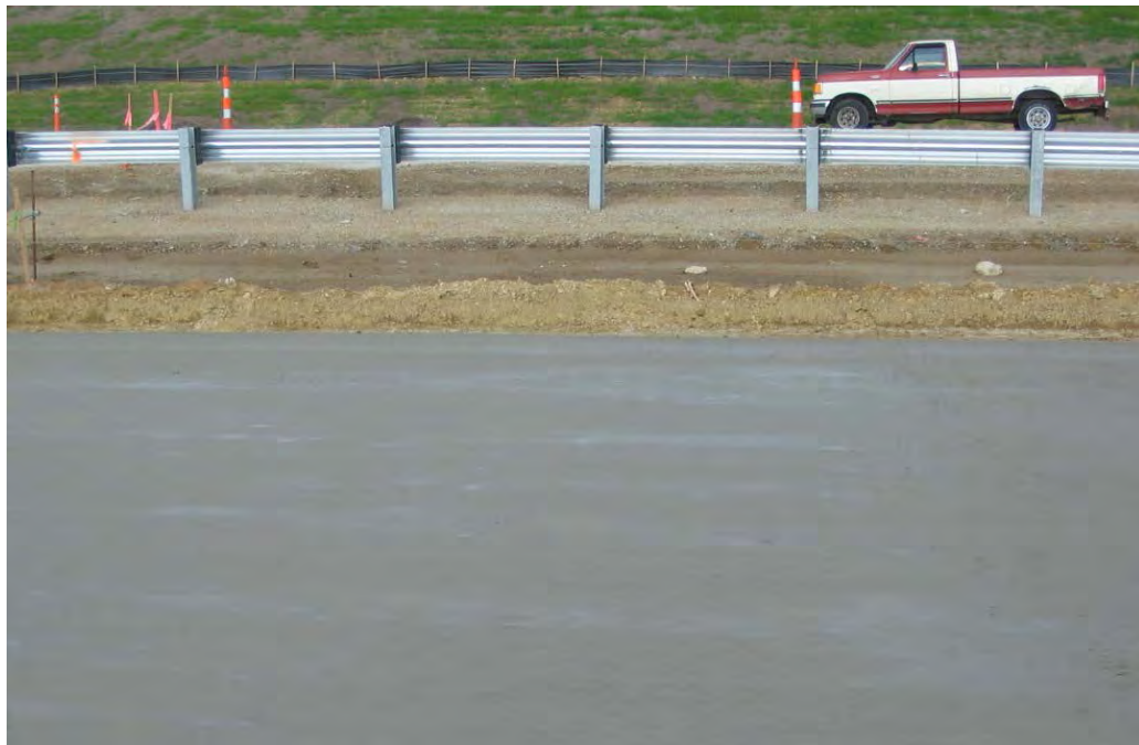
FIGURE 2.2 Bleed Water Rising to Surface After Tining
