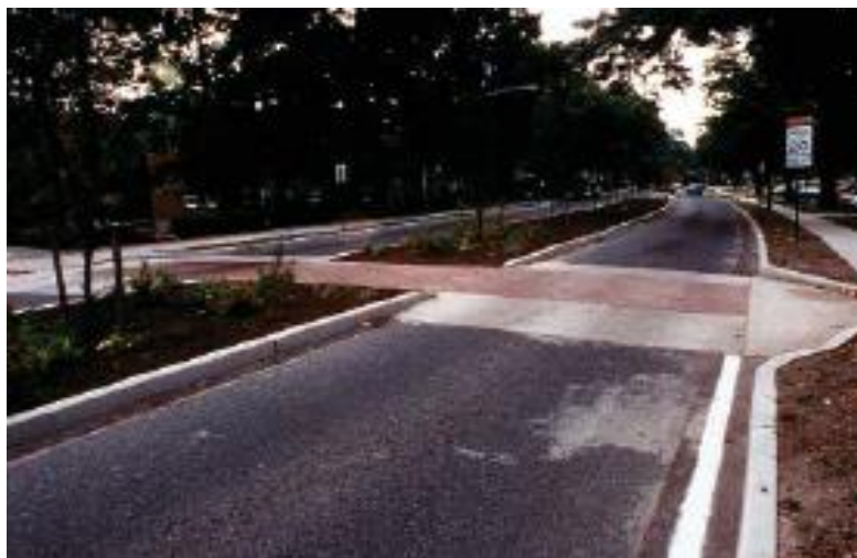
Figure 2-13: Raised Pedestrian Crossing (Harkey and Zegeer, 2004)
