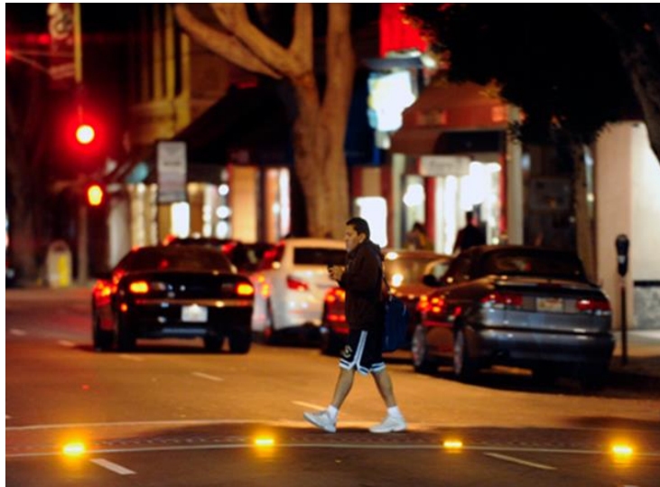
Figure 2-19: Flashing Pedestrian Crossing Lights (McNally, 2012)
