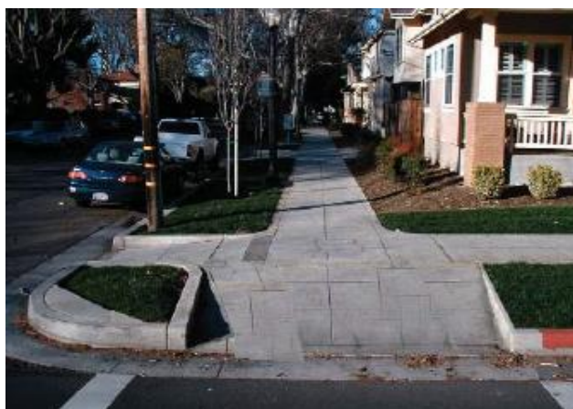
(a) Example of Tight Turning Radii
