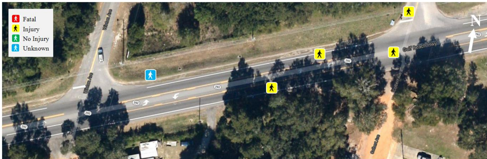
Figure 7-14: Gulf Bch Hwy near Colbert Ave in Pensacola (Roadway ID 48050000; MP 15.737) ( Map )
